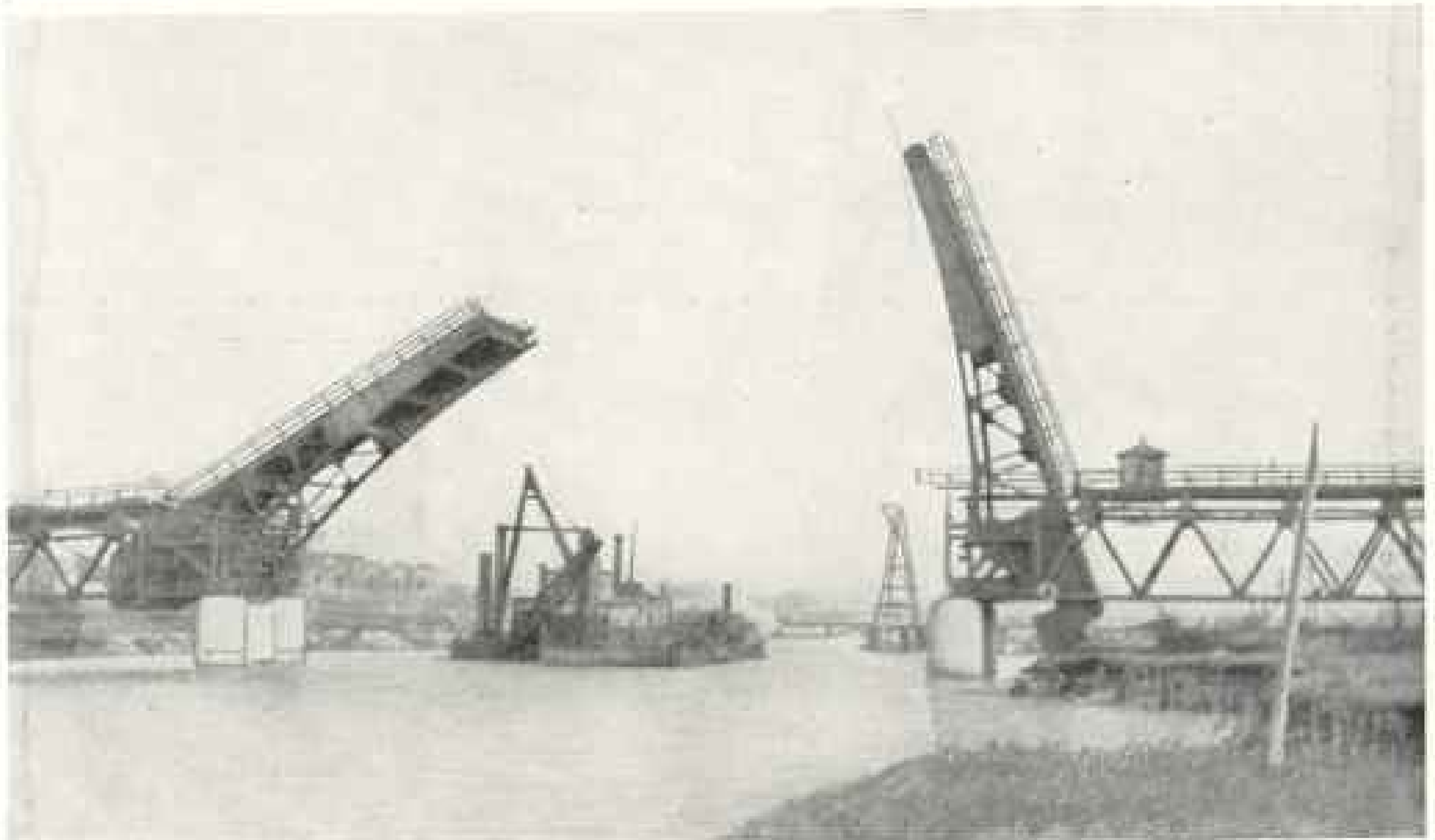
THE HIGHWAY BRIDGE AT SAGAMORE OPEN, ON THE CAPE COD CANAL
