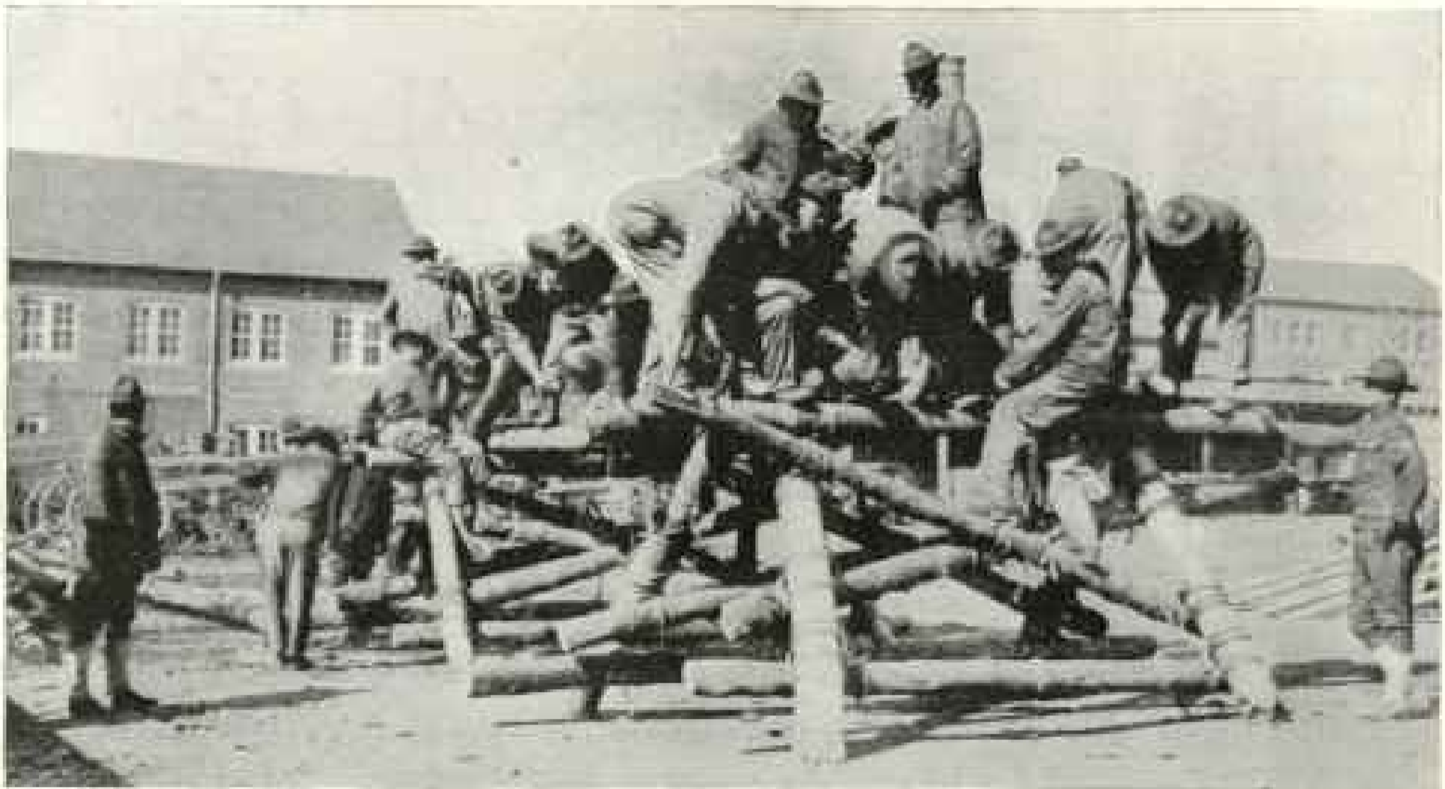
CLASS IN RAPID BRIDGE CONSTRUCTION
