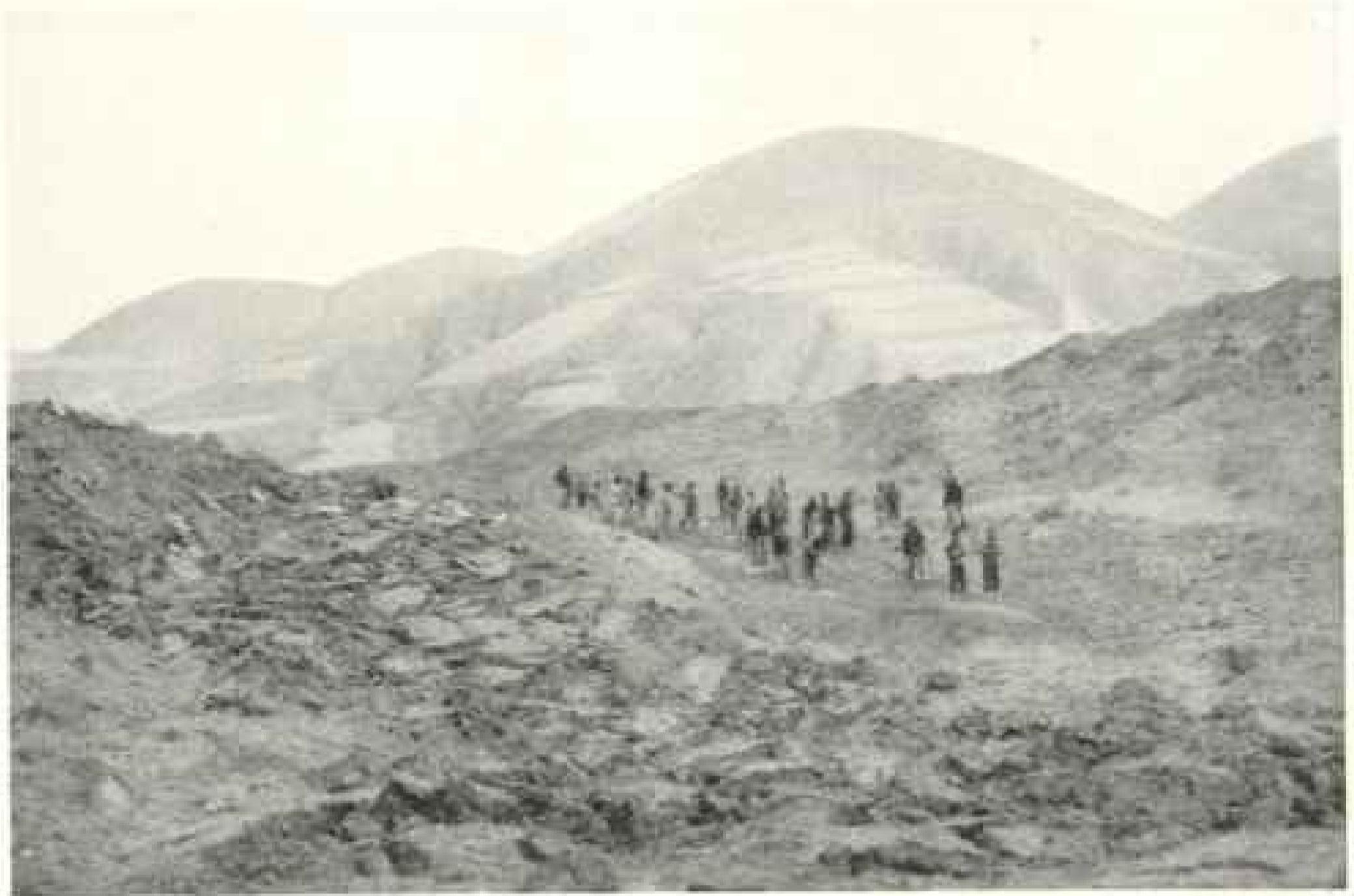
RELIEF WORKERS DIGGING TO RELEASE WATERS BEHIND A QUAKE-MADE DAM The earthquake made this dam of millions of tons of loose earth, stretching from valley-side to valley-side, in a few seconds of time.
