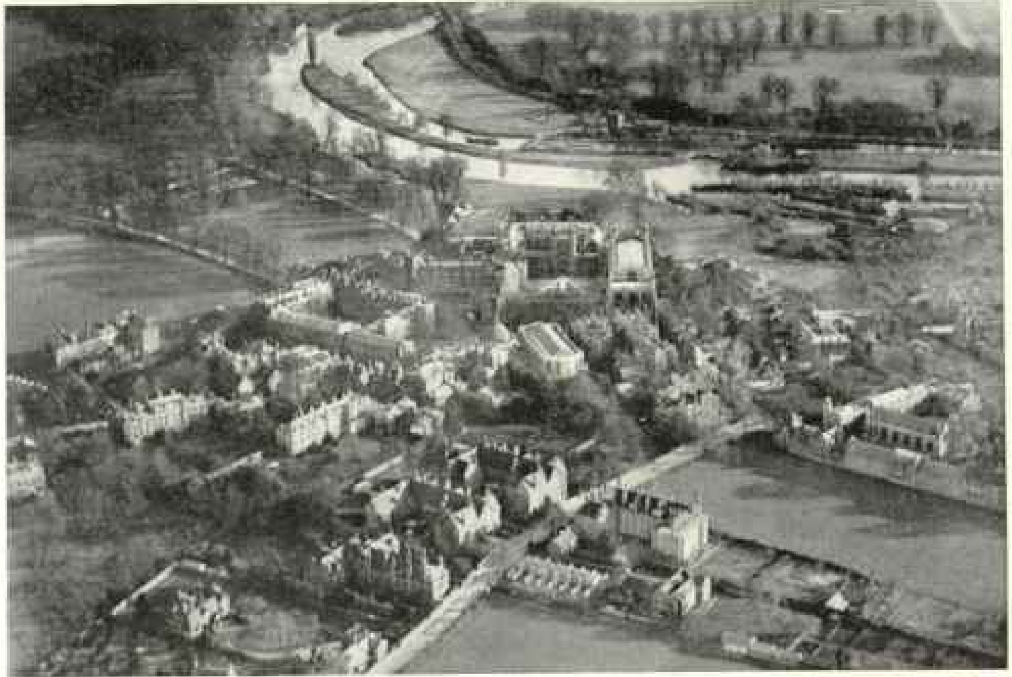
Photograph from Acrofilm, Ltd.
