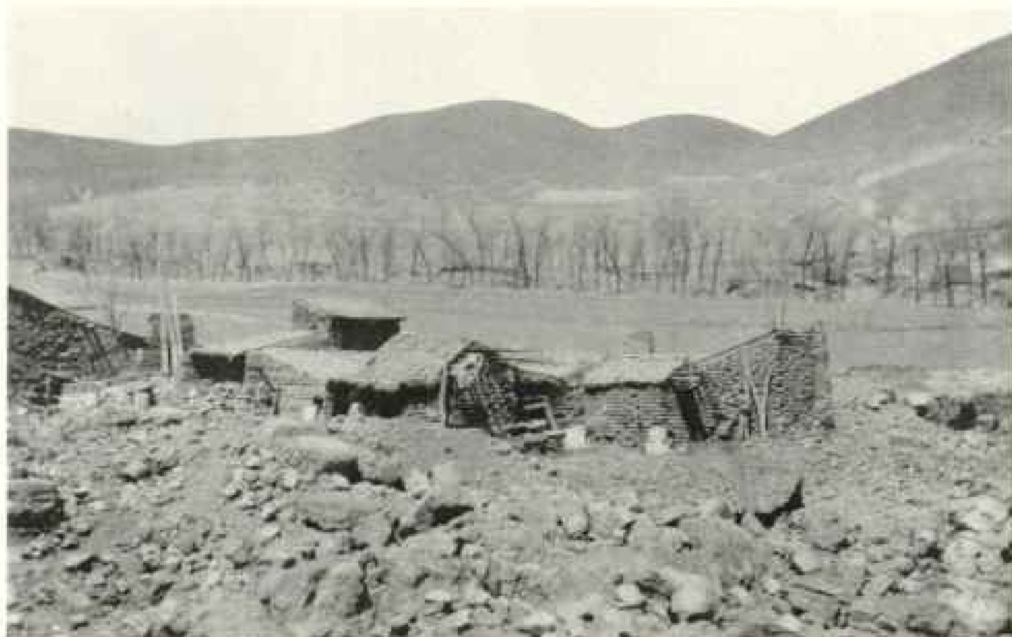
AT THE FOOT OF A SLIDE WHICH BURIED A VILLAGE ON THE VALLEY FLOOR
