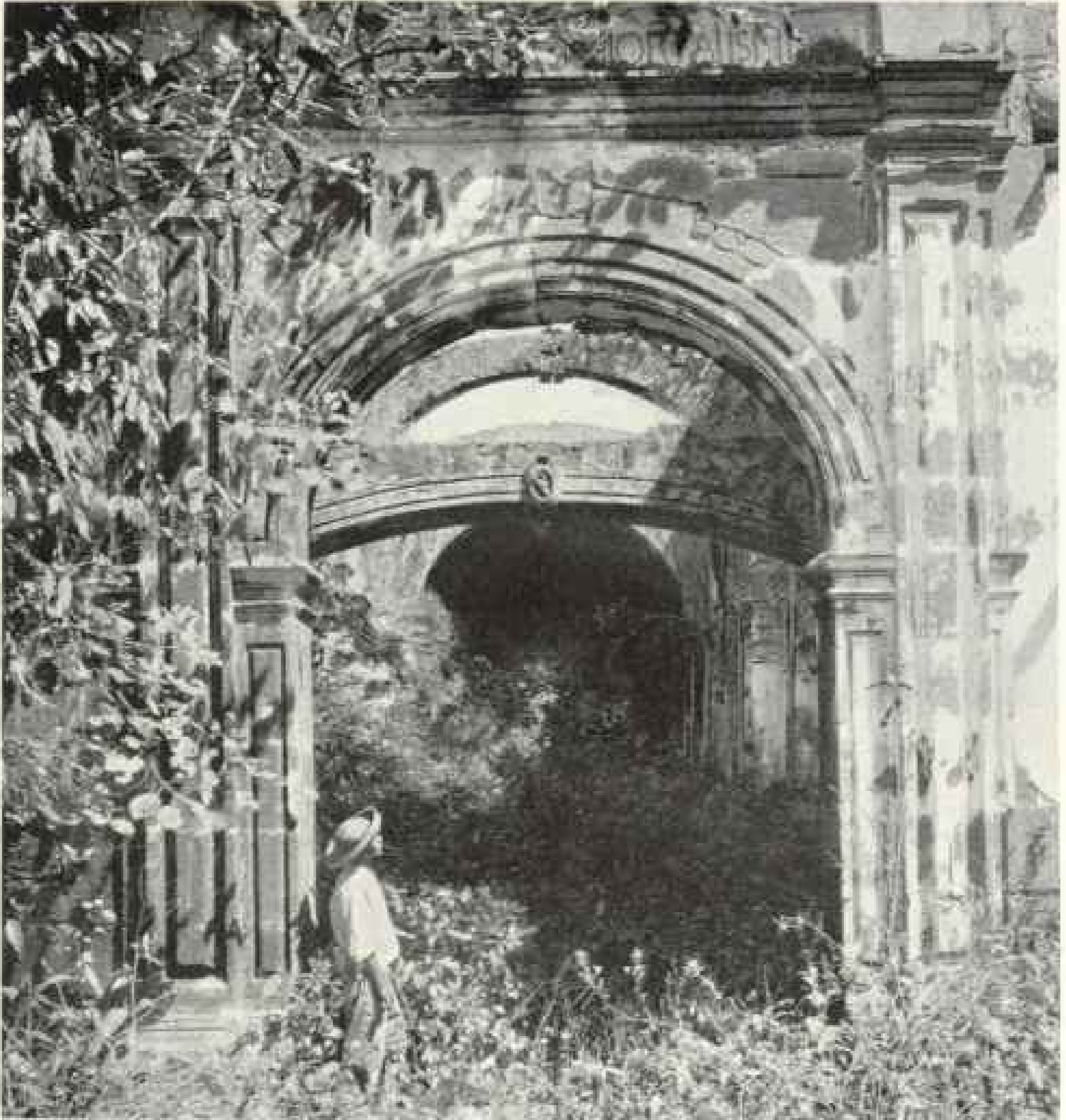
ONE OF THE FINEST EXAMPLES OF A FLAT ARCH EXISTANT IN MEXICO
