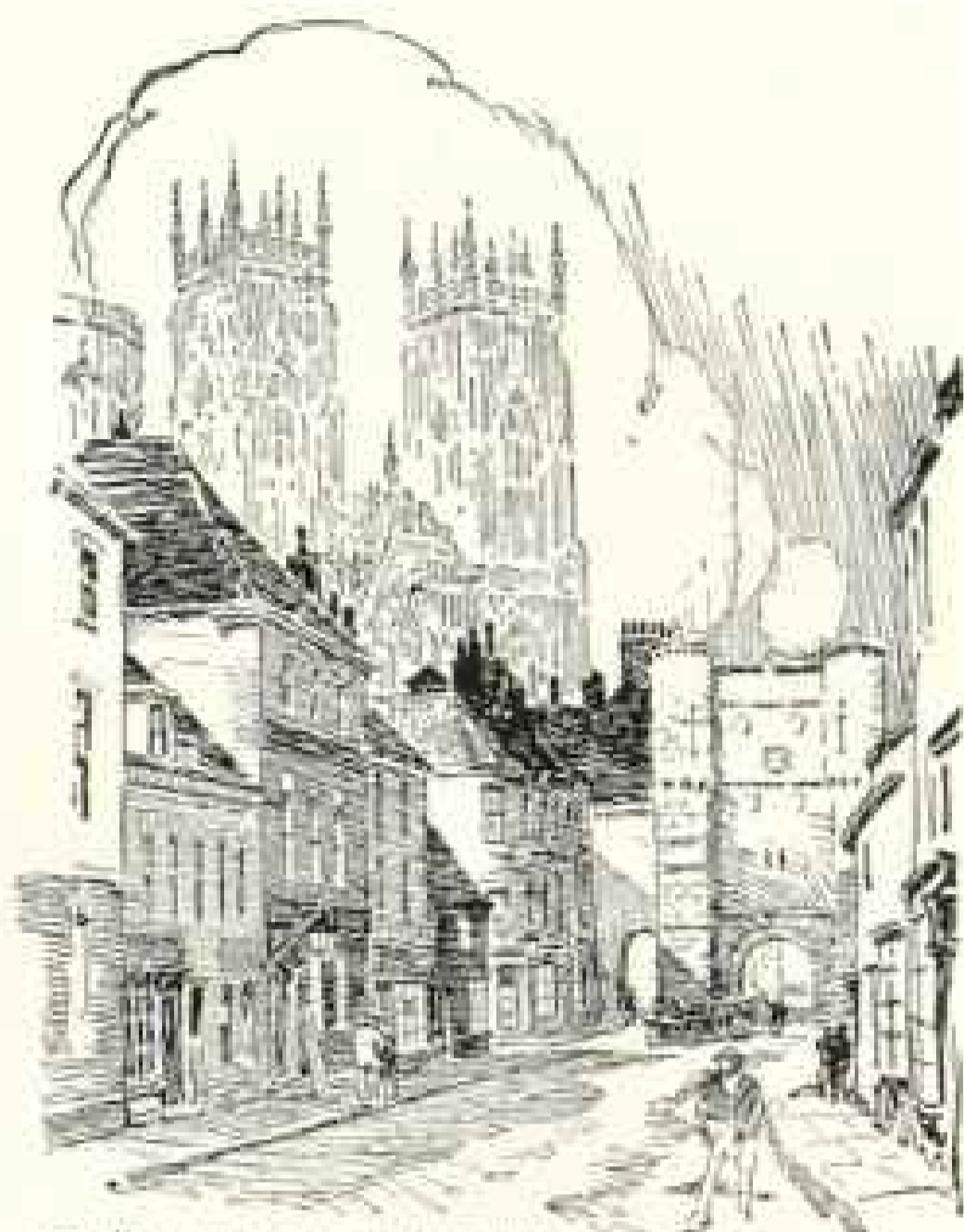
York, "the walled city of great antiquity" on the London and North Eastern Railway
