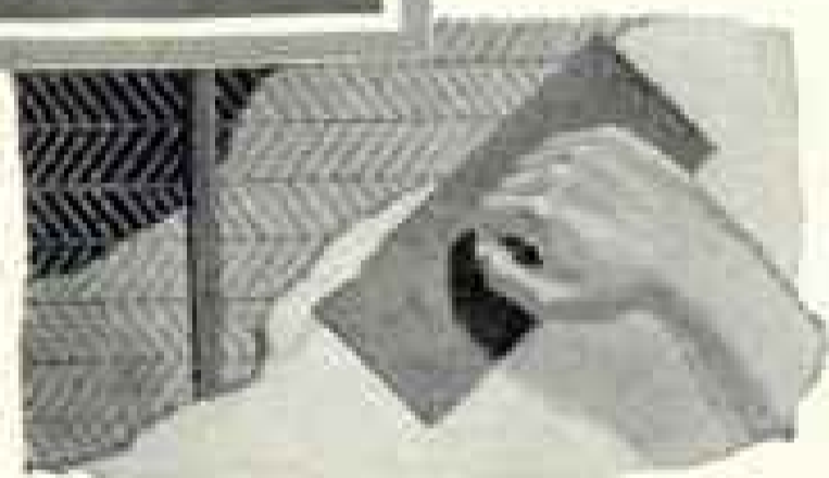
Rigid and durable walls and ceilings, with maximum fire protection and elimination of cracks in plaster, are insured by the use of metal lath made from Sheet Steel.
