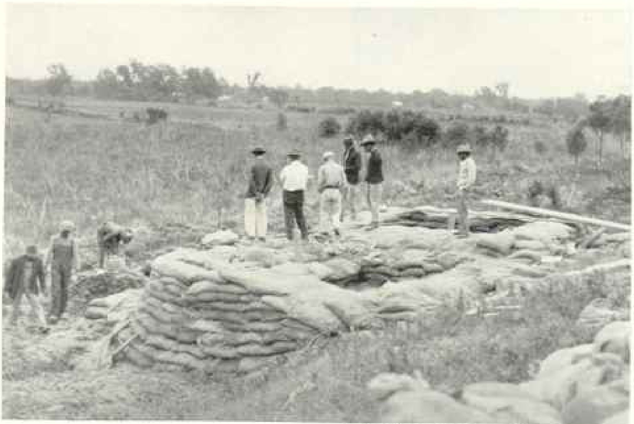
Photograph Courtesy Mississippi River Commission
