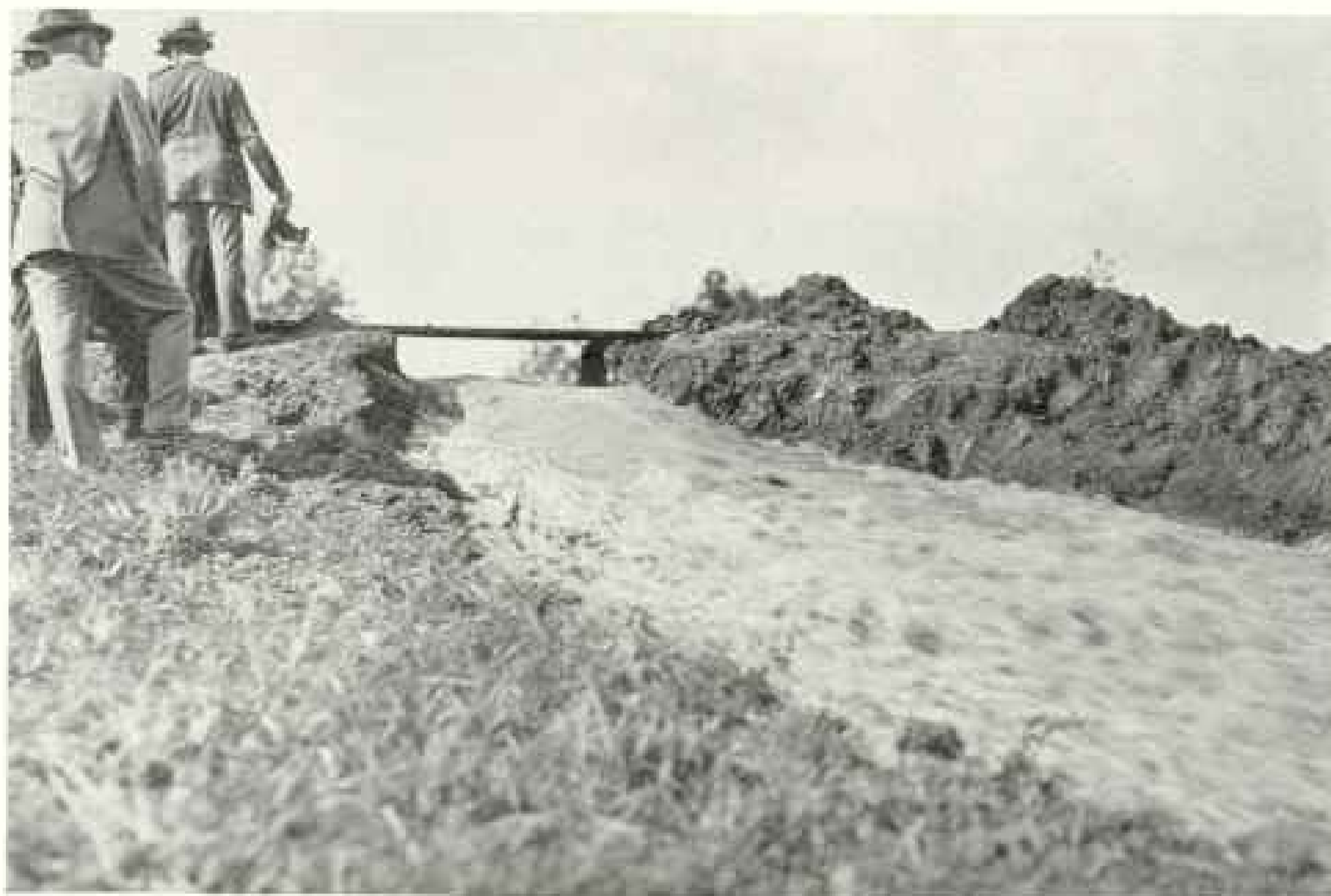
A TINY TRICKLE OVER A LEVEE MAY GROW TO A RAGING TORRENT.
