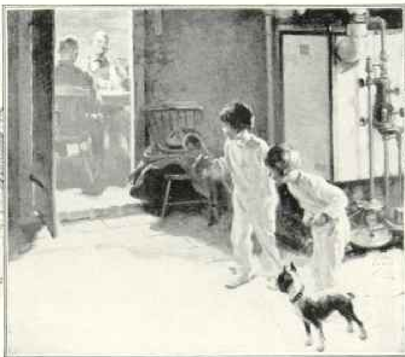
Bryant Gas Heating adds an extra room to the house.
