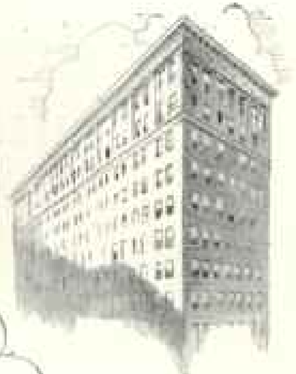
This Office Building at 99 Worth St. is one of many of New York's famous Skitline Te-pe-co equipped.
