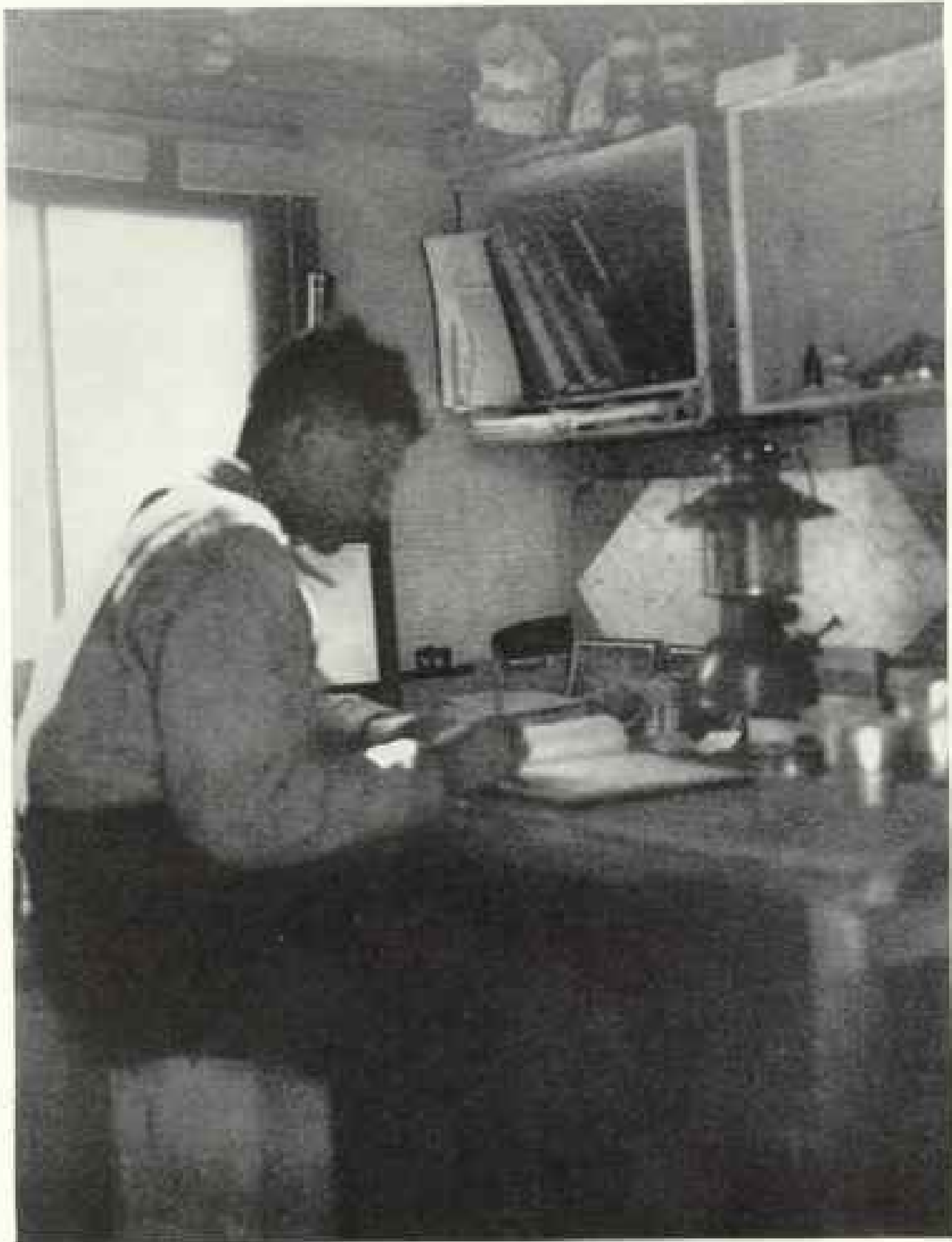
BEARDSLEY AT WORK IN THE "EMPIRE STATE BUILDING"
