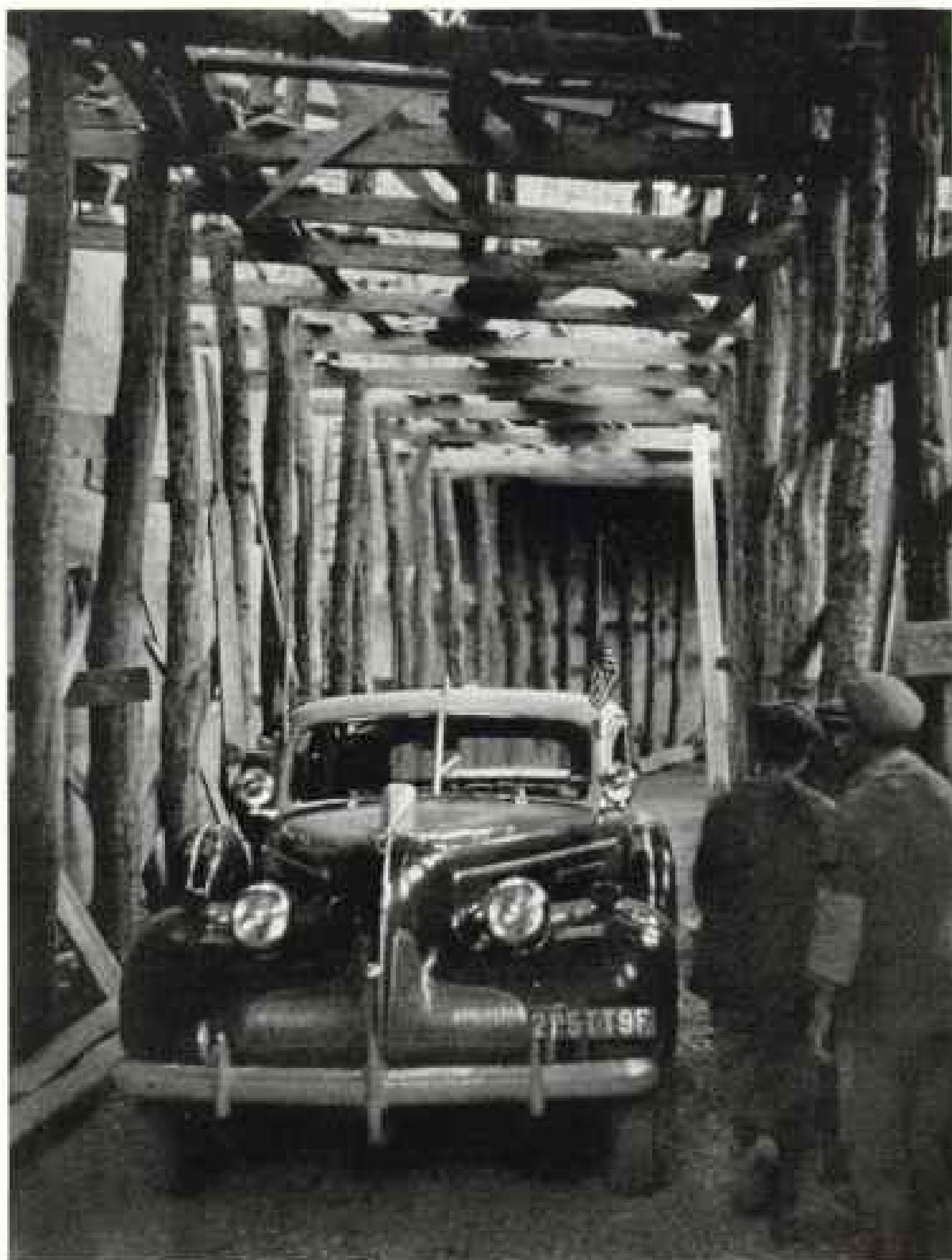
A Tunnel Was Under Construction at the Top of the Chalus Road
