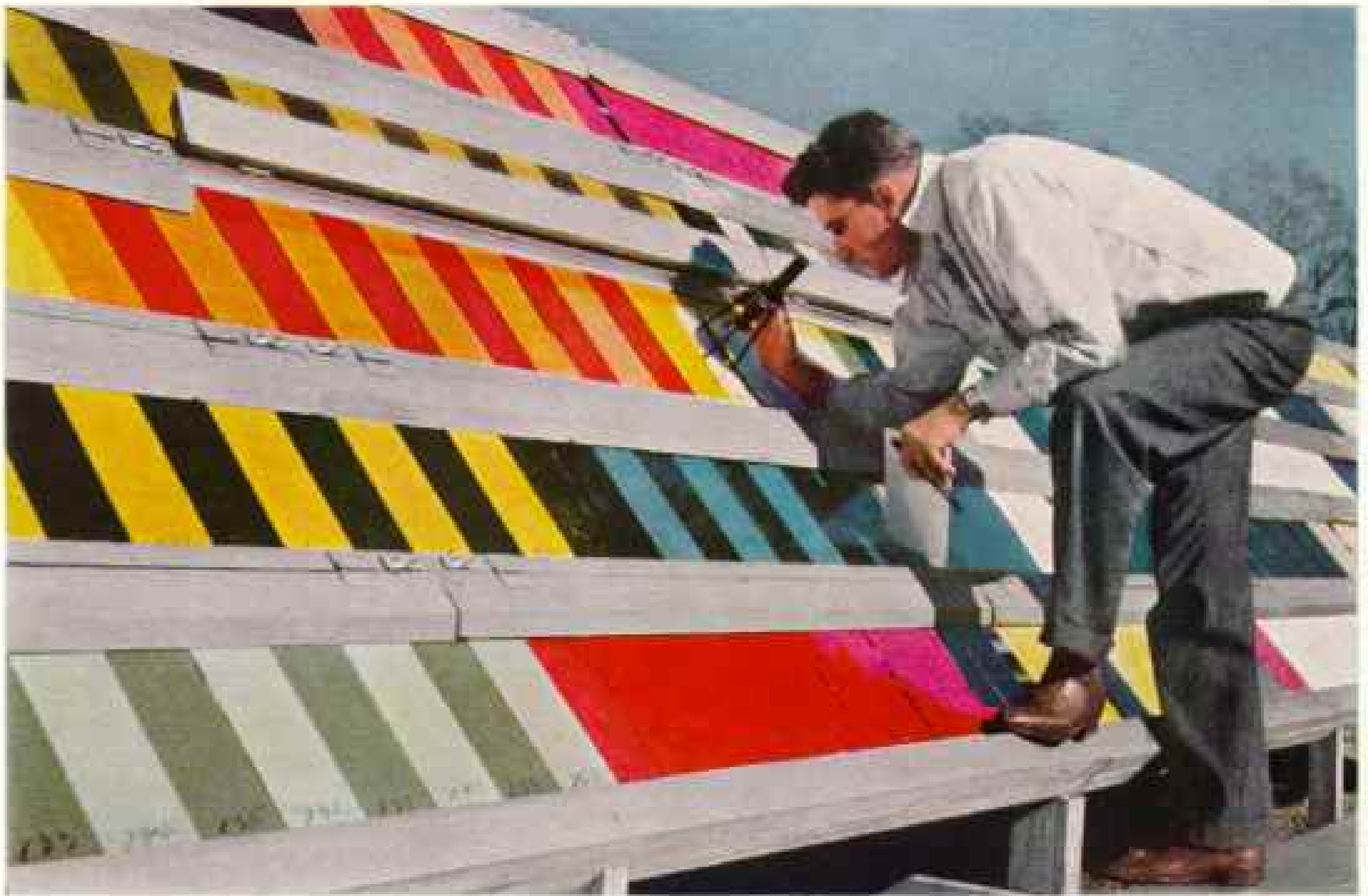
Paint's Durability Is Tested by Exposure to All-year Weathering
