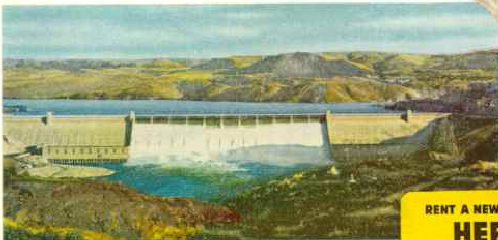
Grand Coulee Dam, only 227 miles from Walla Walla, Wash., is one of the mightiest constructions built by man...550 feet high, 4,173 feet long, 500 feet thick at base, 3 times bigger than the largest Egyptian pyramid. This majestic Dam harnesses the waters of the scenic Columbia River.
