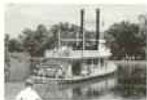
WEST FRONT CITY AND HISTORIC GREENFIELD WALKS
