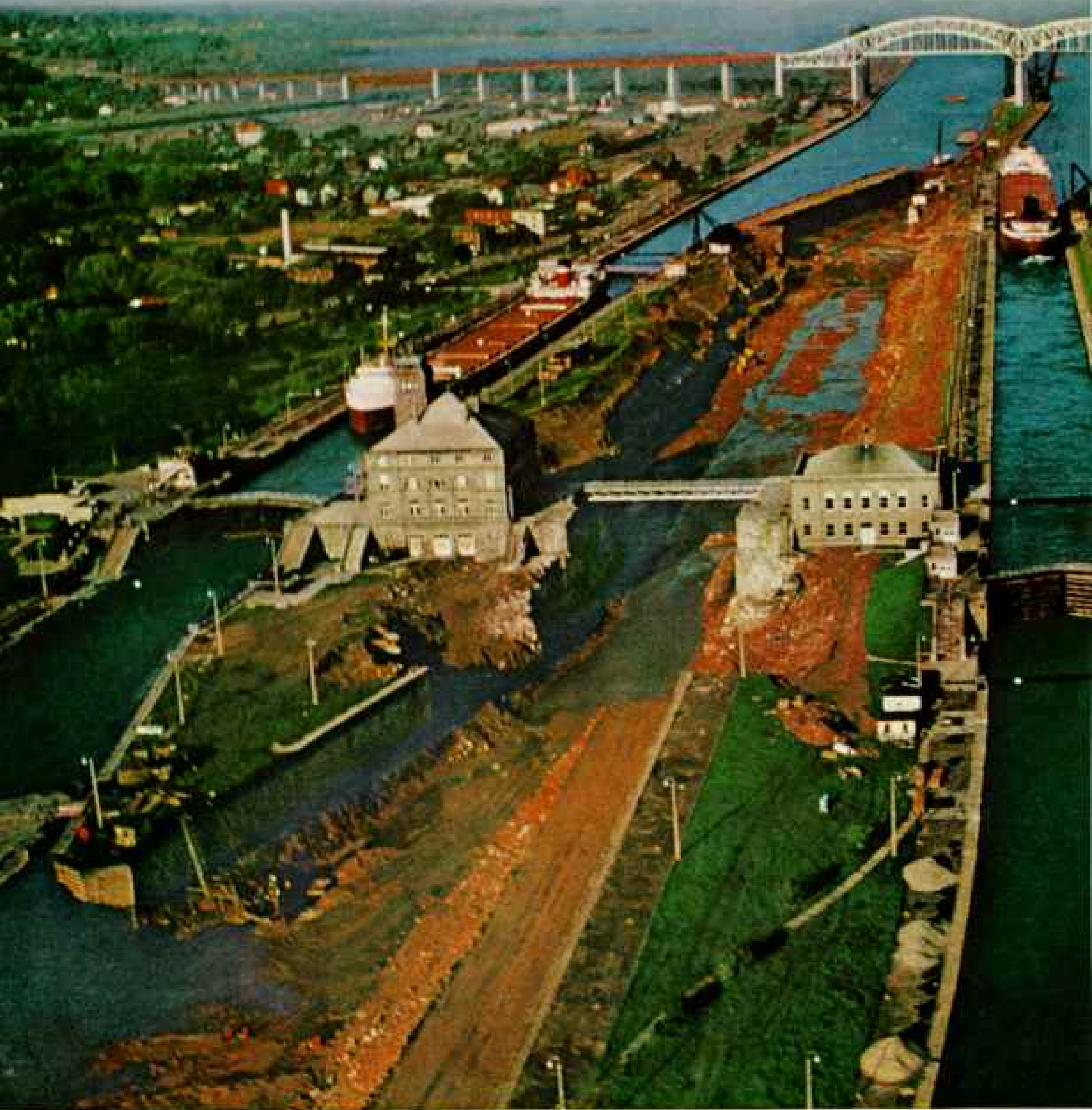
Sault Ste. Marie Locks, in the busy Soo Canal, lift Great Lakes carriers over a 22-foot drop
