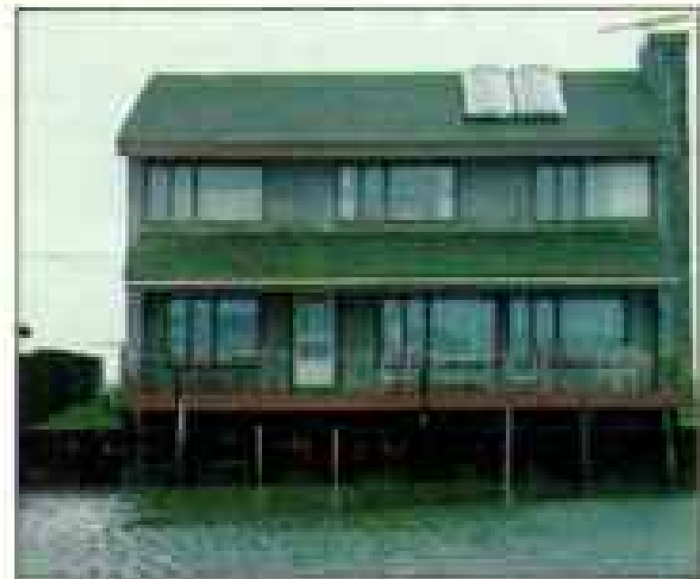
Sunstream solar collectors on the Fiore home in New Jersey.
