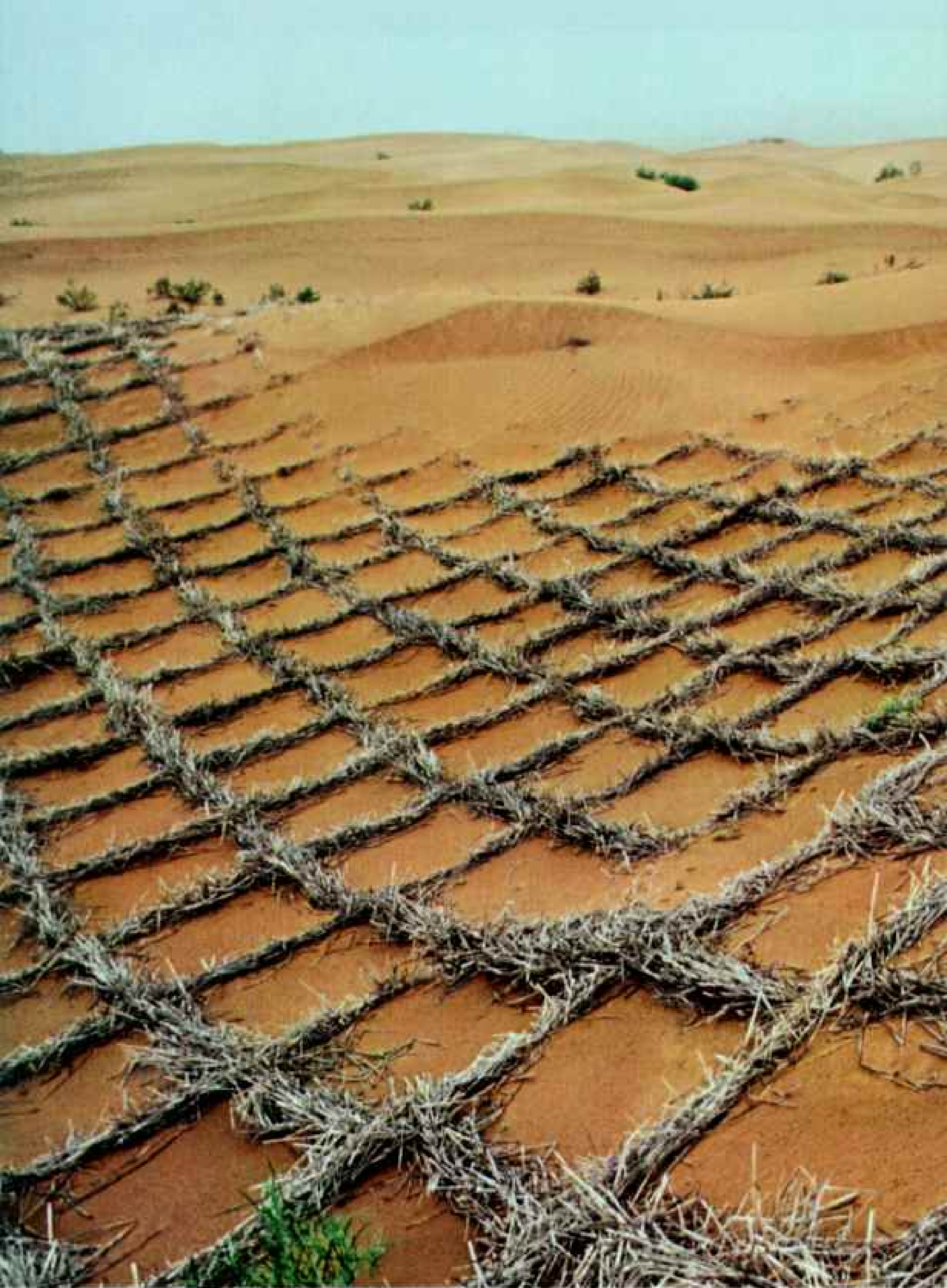
Stemming a tide of sand, a grid of straw checks dunes advancing on a
