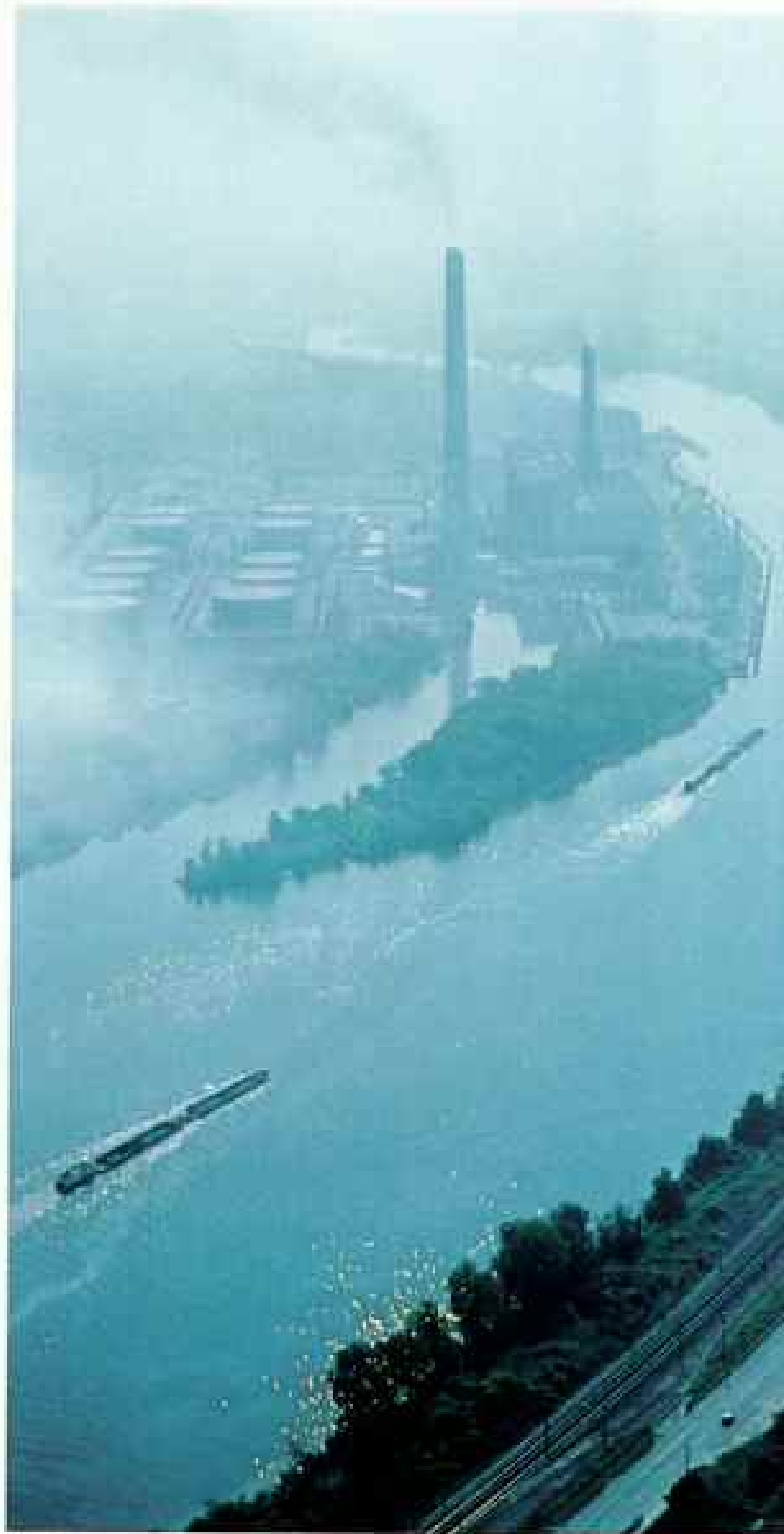
A scrim of smog obscures stacks of the oil- and coal-fired Électricité de France generating plant at Porcheville. Upstream, construction has begun on a nuclear power plant at Nogent to provide 5 percent of the country's power by 1987.
