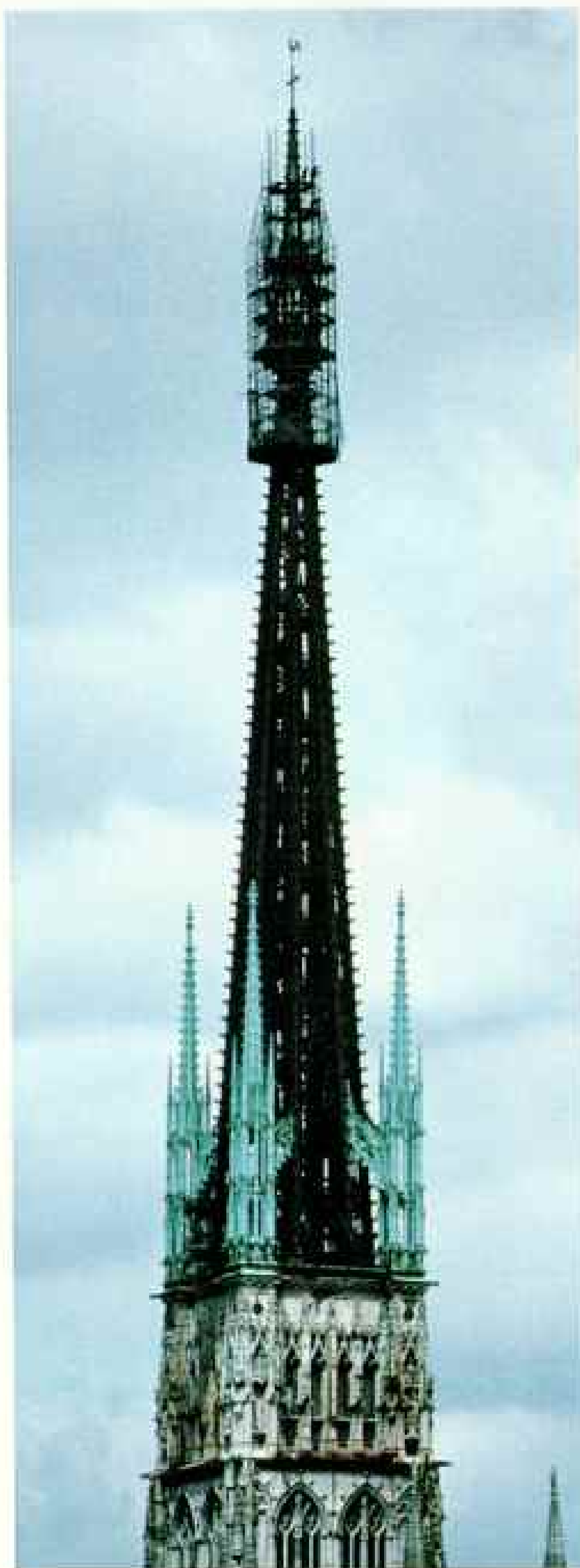
With heavenly aspirations, a 495-foot-high spire soars above the Cathedral of Rouen (above), damaged by Allied bombs during World War II. Workers engaged in renovations scale a scaffold (right) wrapped around the cast-iron spire, a 19th-century addition to the cathedral.
