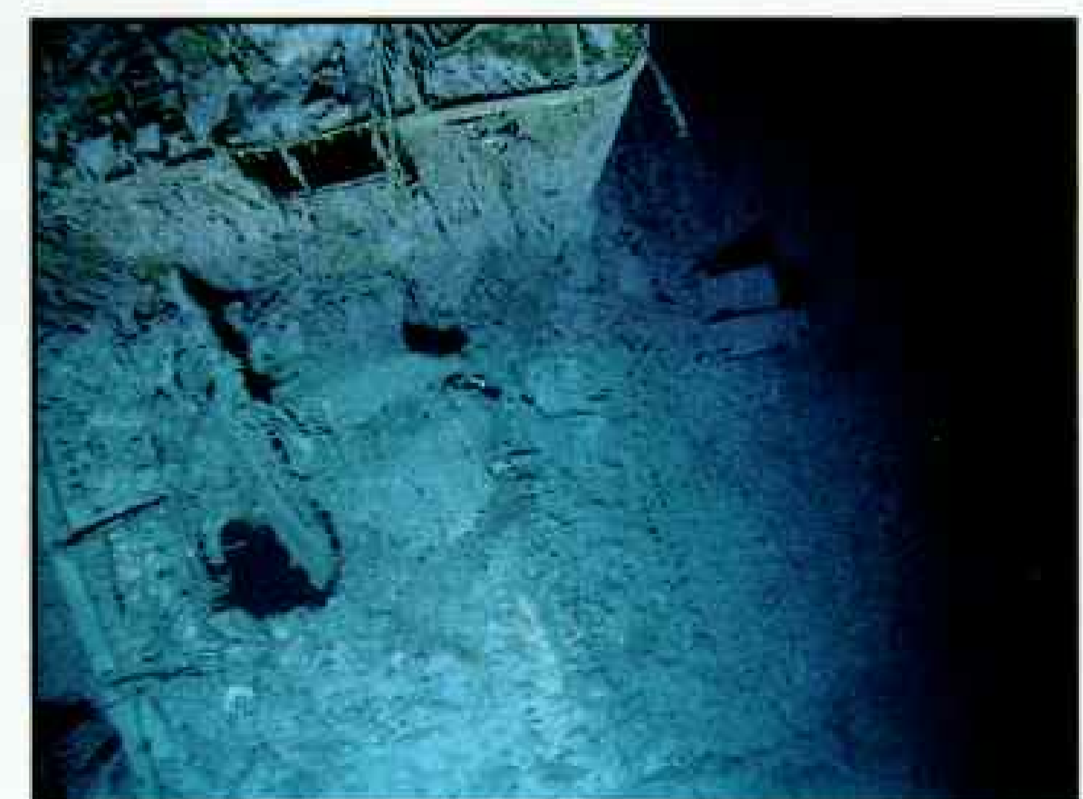
9 Opening for air duct, top, overlooks hole in the roof of the first-class reading room.
