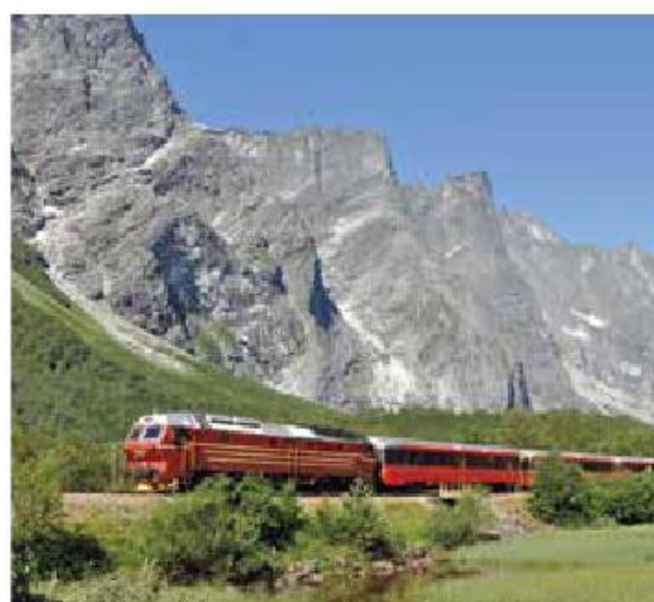
The towering rock face of Trollveggen juts high above the Rauma Railway.
