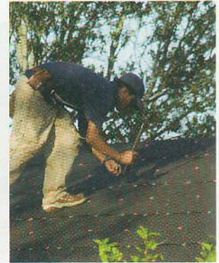
▲ fix the roof
