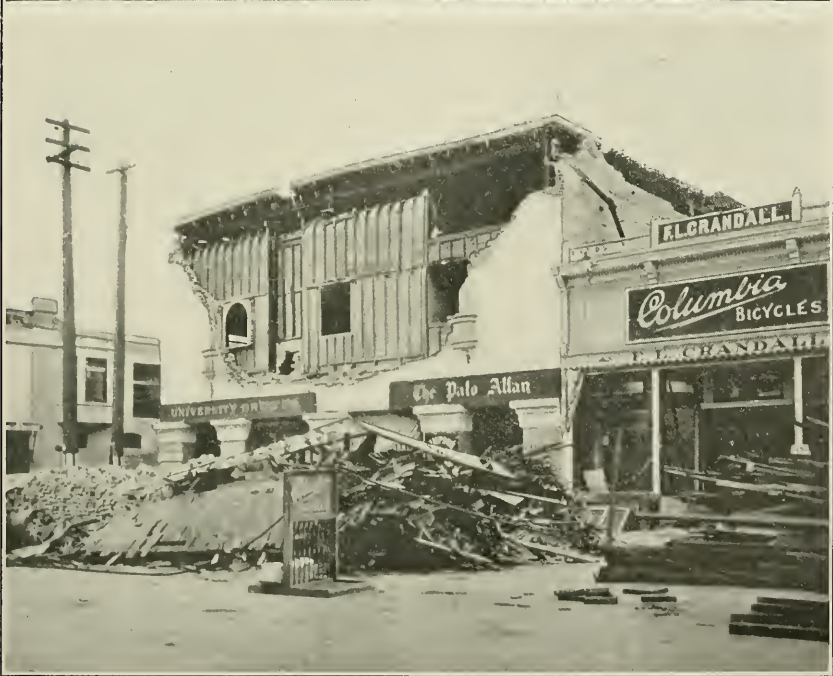
Photos by W. C. Mendenhall, U. S. Geological Survey Scenes at Palo Alto. Opposite the depot. A Wrecked Building on University Avenue
