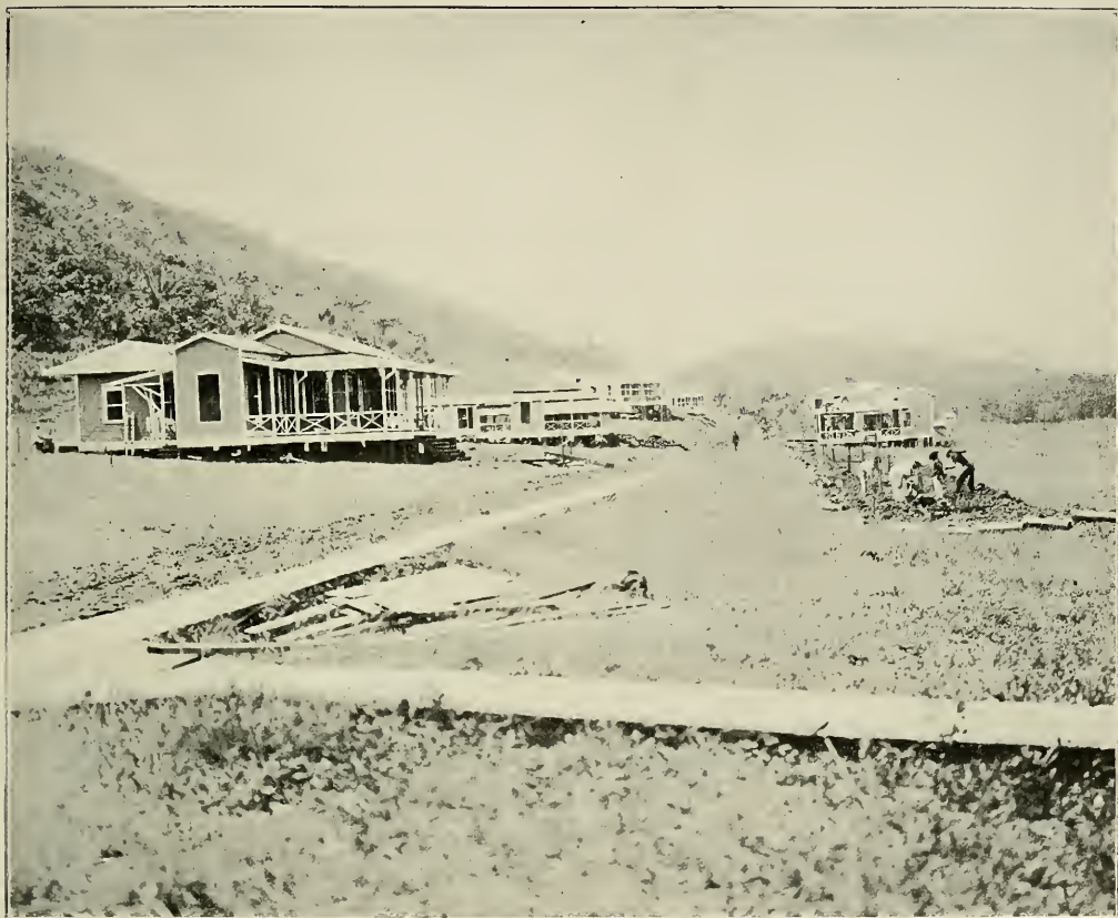
Cottages for Married Employees, at Corozal
