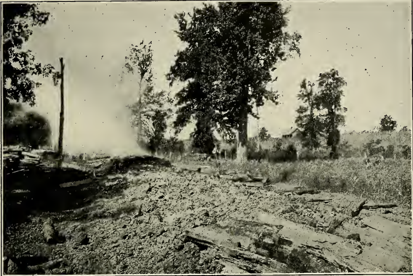
One Section of Road Burned and a Second Section Being Fired
