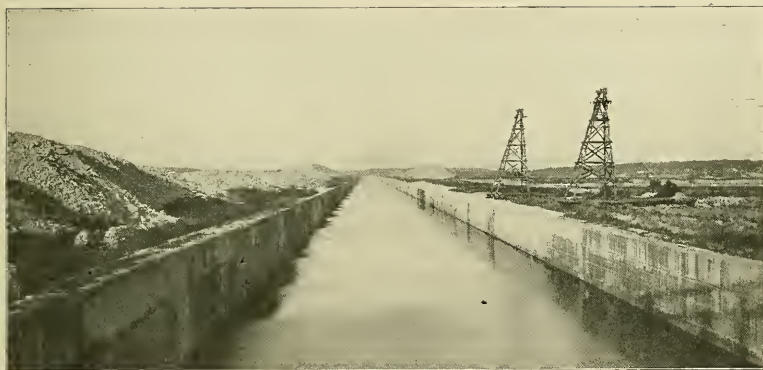
A View of the Chicago Drainage Canal
