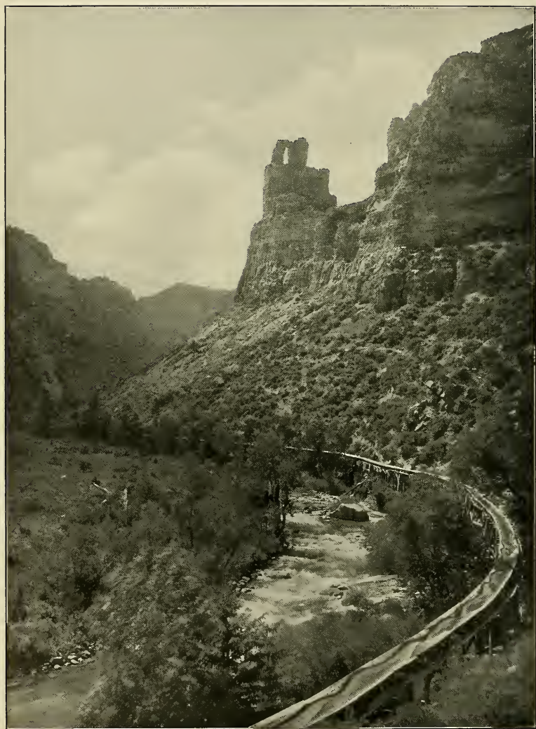
Looking up the Canyon of Tongue River on the East Side of Bighorn Mountains Walls of limestone with typical castellated structure; shows flume in which railroad ties are floated from the central mountains to the plains
