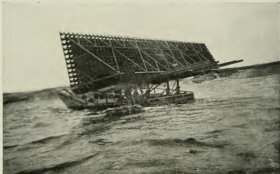
THE CYGNET SAFELY LIFTED ON TO ITS RAFT AND READY TO BE TOWED HOME
