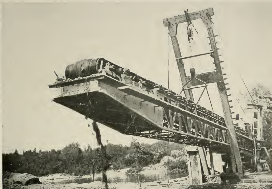
TYPE OF CONVEYOR DREDGE USED IN CHANNEL-DEEPENING
