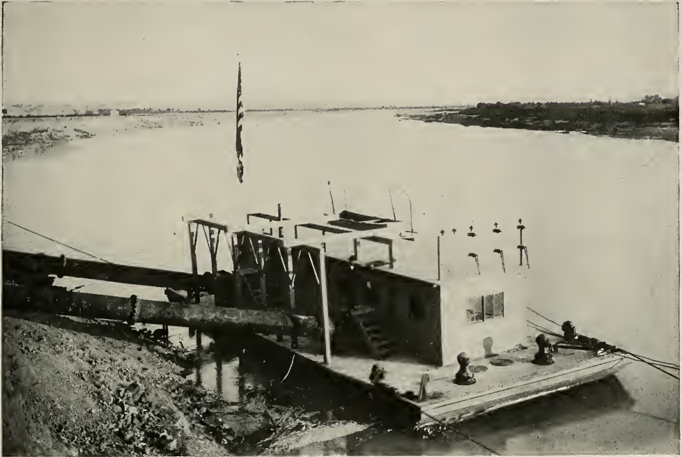
PUMPING BARGE OF THE U. S. RECLAMATION SERVICE: WILLISTON PROJECT, NORTH DAKOTA (SEE PAGE 252)
