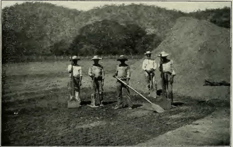
PROVIDED WITH WOODEN SPADES THE PEONES GATHER THE SALTED EARTH INTO LONG, NARROW HEAPS
