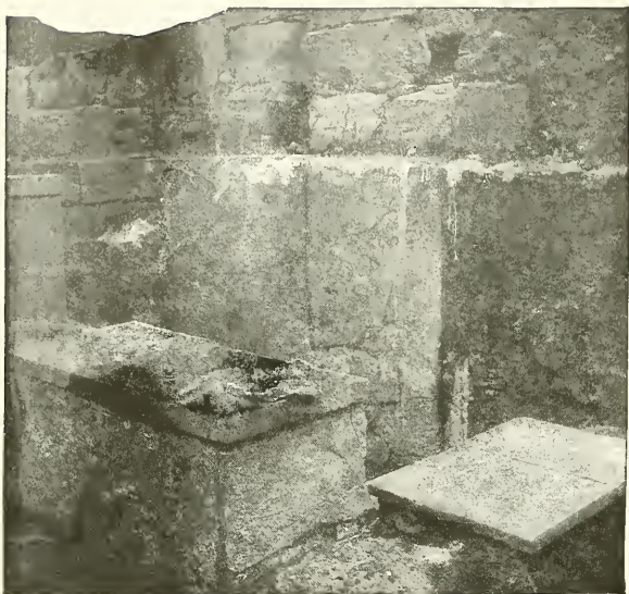
A BATHROOM IN THE PALACE OF KNOSSOS
