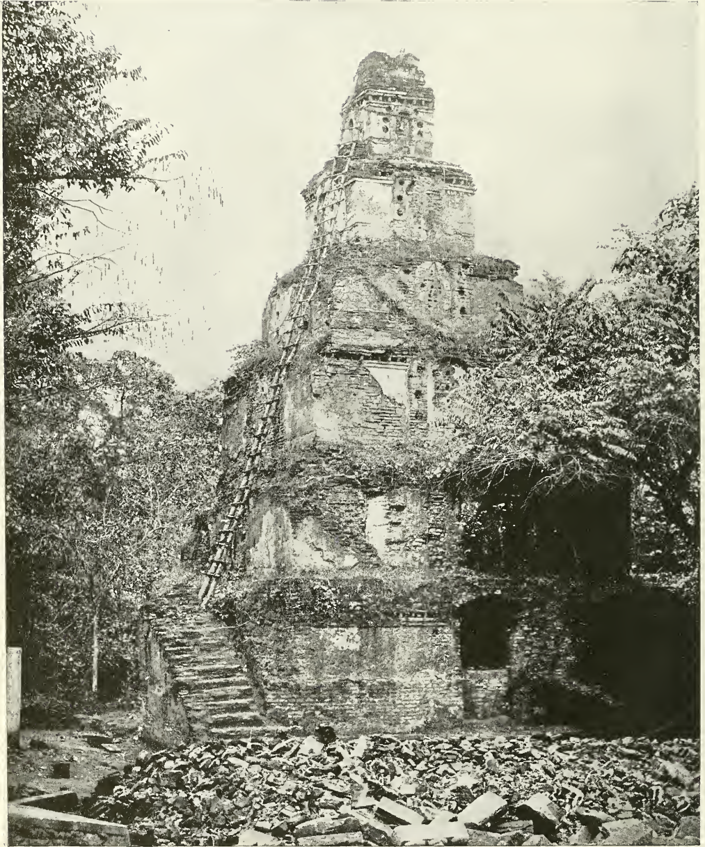
THE PALACE OF SEVEN STORIES, OR SAT-MAHAL-PRASADA, AT POLONNARUWA Its origin and purpose are unknown. An outer staircase leads to the second terrace only; inner staircase to second level only
