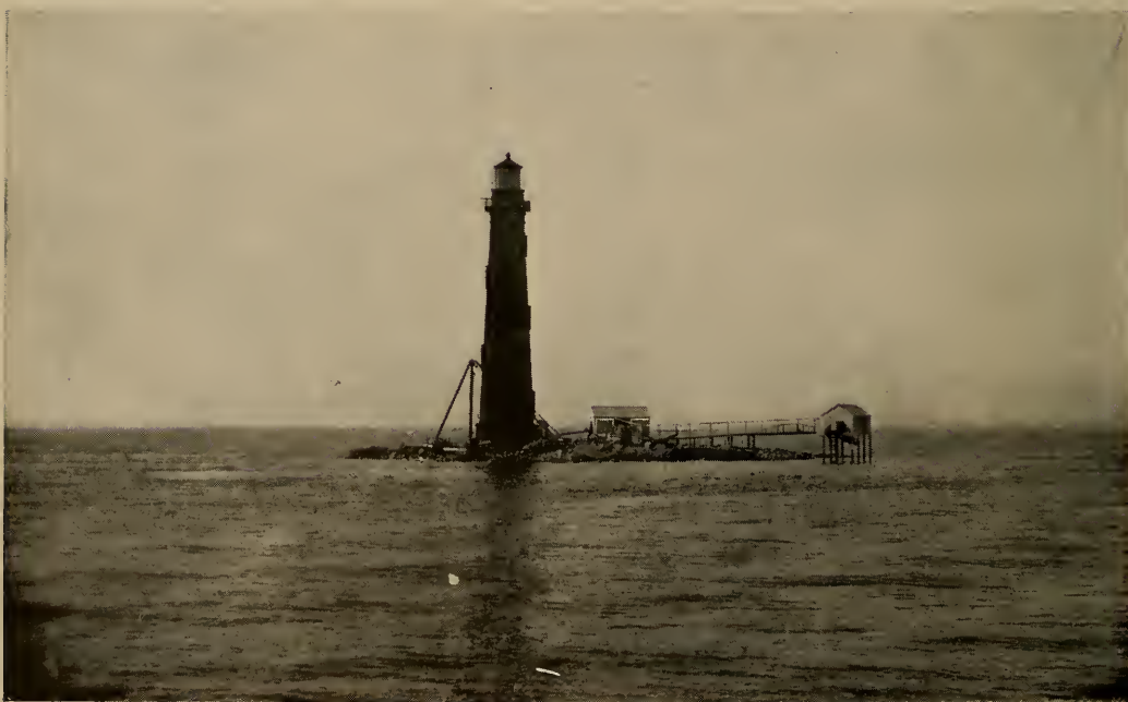
THE SAND ISLAND LIGHT STATION AFTER THE HURRICANE
