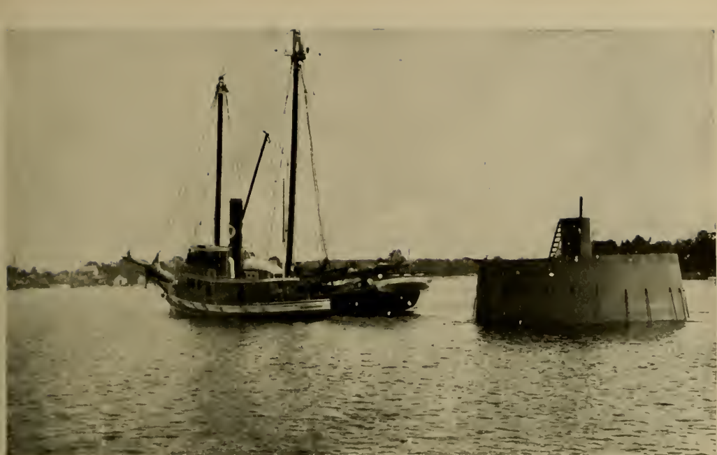
A TUG TOWING A CAISSON TO BE SUNK FOR A LIGHTHOUSE FOUNDATION (SEE PAGES 20 AND 26)
