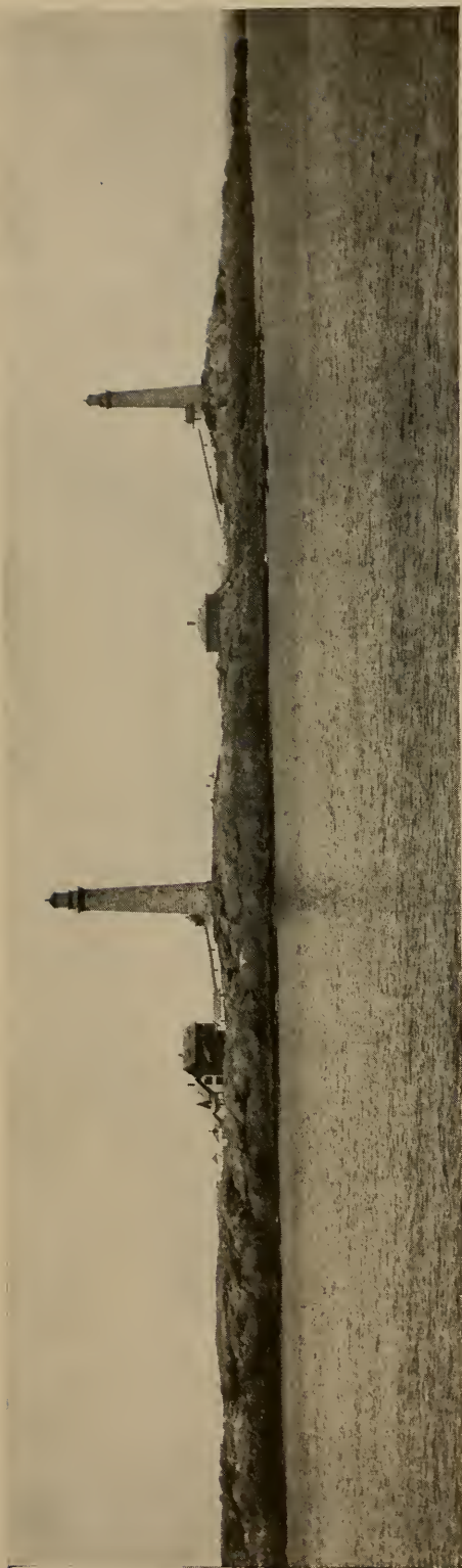
THE TWIN LIGHTS OF CAPE ANN, MASSACHUSETTS Two granite towers, originally built in 1789. The two fixed lights were established to furnish a distinctive aid, a purpose which now would be attained by a single flashing light (see pages 27 and 37)
