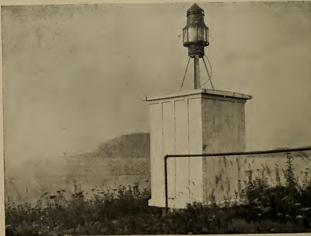
A LIGHT WHICH FLASHES EVERY 3 SECONDS FOR 5 MONTHS WITHOUT ATTENDANTS Many such lights have been installed to mark the inside passages in Alaska. This one is placed at Point Retreat, Alaska
