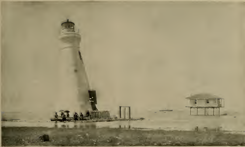
THE CHANDELEUR LIGHT-TOWER, LOUISIANA, WHICH WAS ABANDONED AFTER BEING UNDERMINED BY A TORNADO IN 1893
