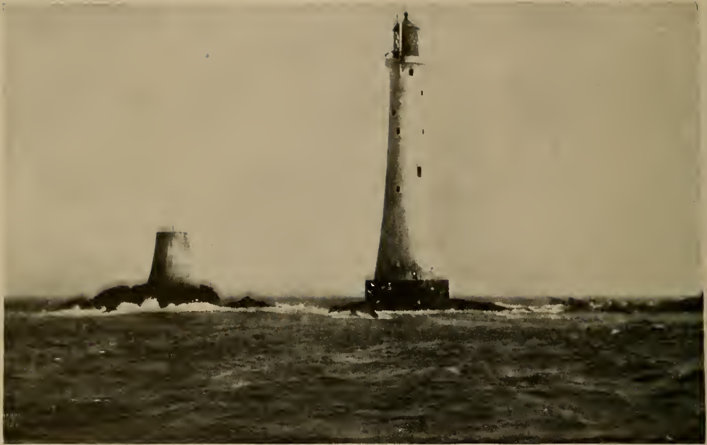
THE FOURTH AND PRESENT EDDYSTONE LIGHTHOUSE, COMPLETED IN 1881 (SEE PAGE 17)
