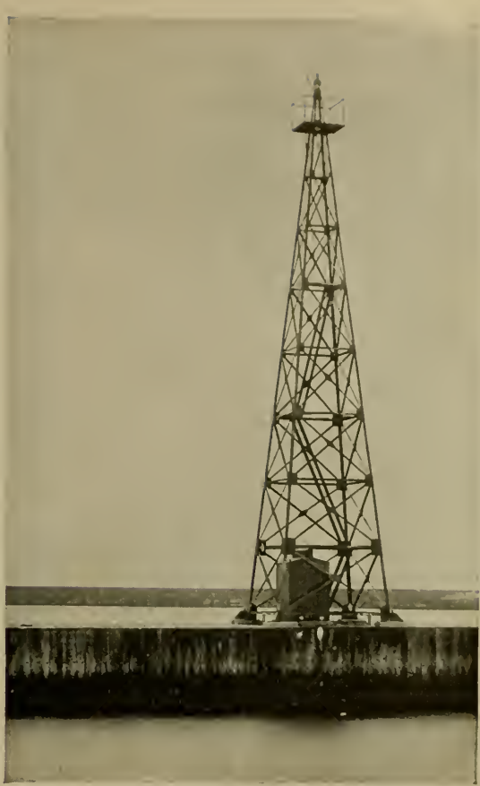
AN ACETYLENE GAS LIGHT, THE FAIRPORT WEST PIER LIGHT, OHIO
