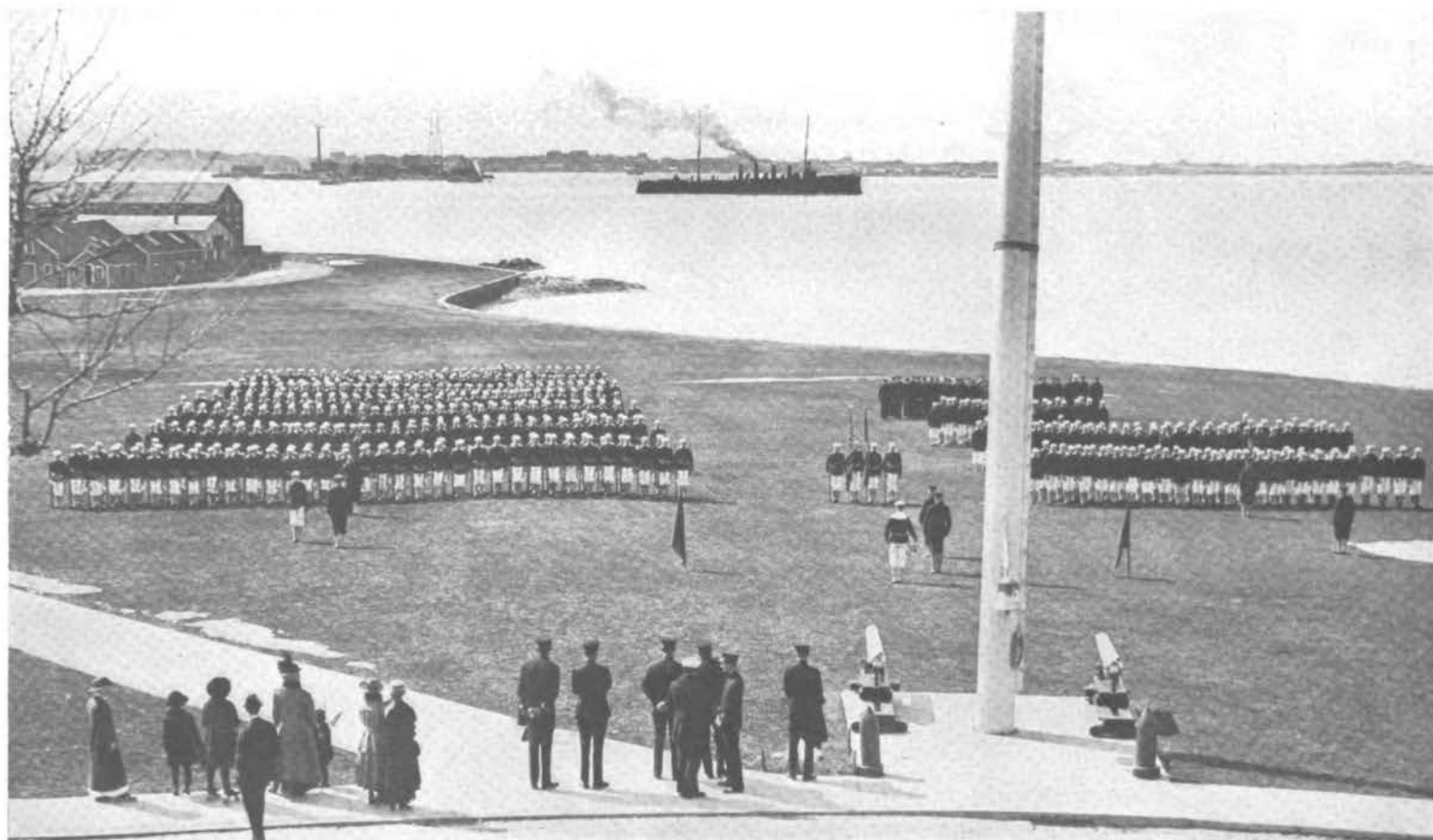
LINED UP FOR INSPECTION
