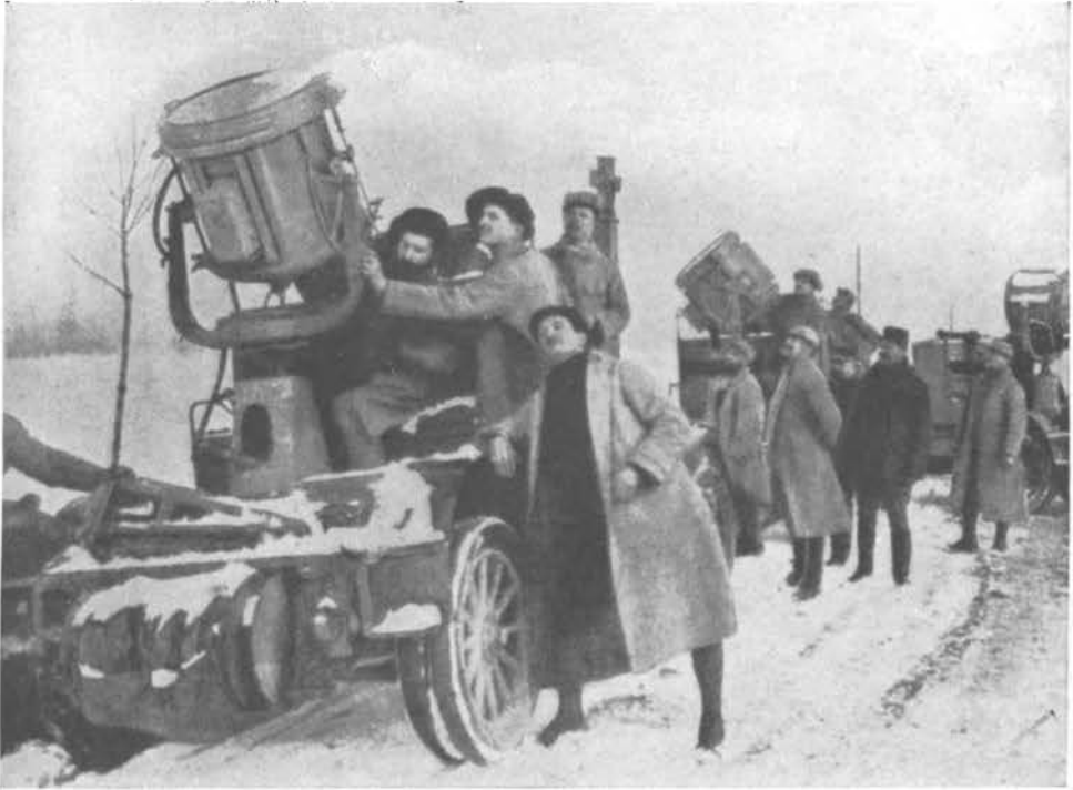
THE AUTOMOBILE SEARCHLIGHTS WHICH ARE MOST EFFECTIVE IN SEARCHING OUT THE ENEMY'S ZEPPELINS, THUS AIDING IN BRINGING THEM DOWN
