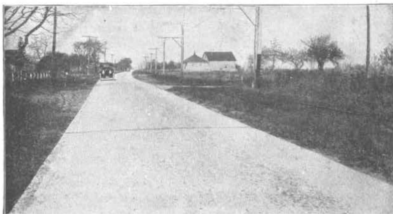
Lake Shore Concrete Road Near Kenosha, Wis., Built for the State Highway Department by G. R. Wade, of Kenosha, in 1915
