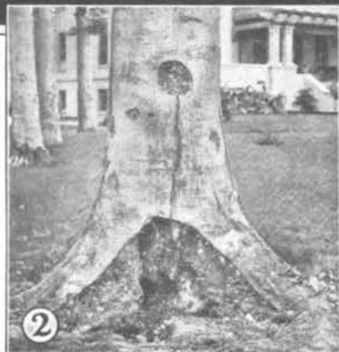
2 Cement patch removed—showing extensive and neglected decay.
