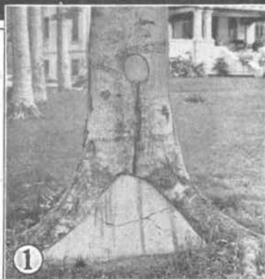
1 A crude cement patch—ineffective and injurious.
