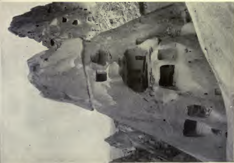
IN MANY CONES THE EXTERNAL WALLS THEMSELVES HAVE ROTTED AWAY, LEAVING THE CHAMBERS EXPOSED
