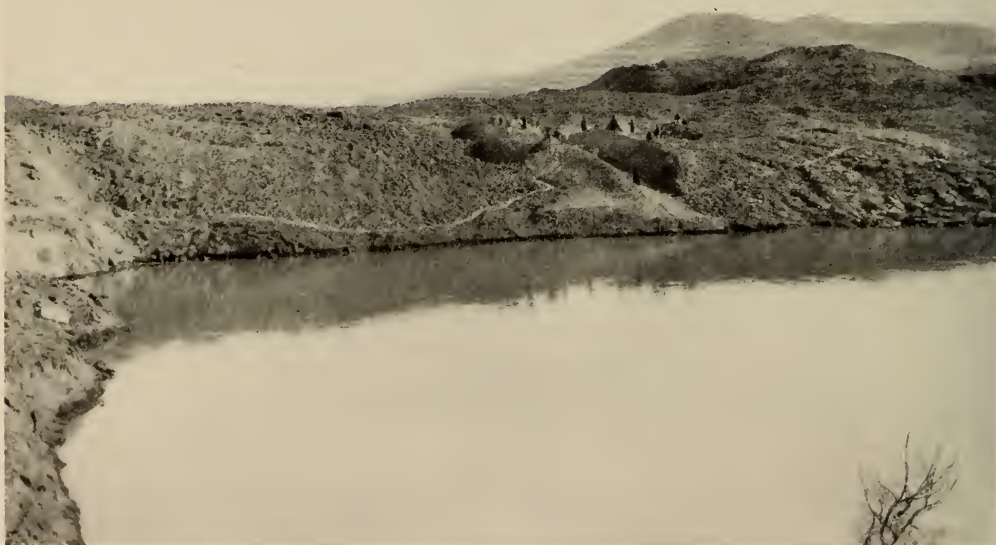
A MOUNTAIN STREAM DAMMED UP BY A LANDSLIDE OUT OF THE HILLS Excavators are seen in the background working to release the waters which have formed a lake. The water is likely to break through the loess at unexpected places and times.
