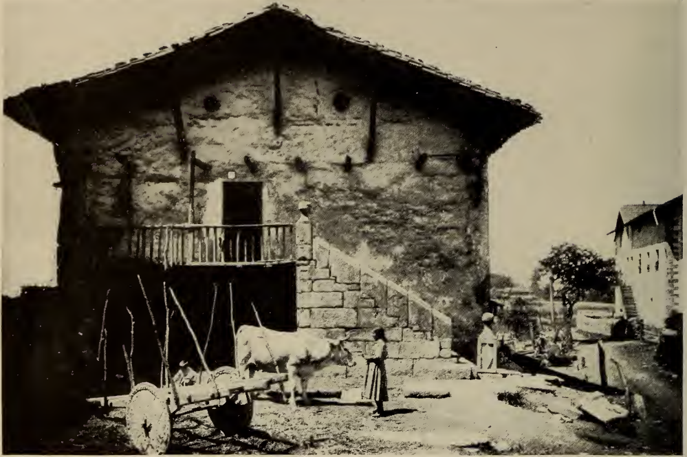
A TYPICAL, BASQUE FARM-HOUSE, WITH A HEAVY TWO-WHEELED CART IN THE FOREGROUND
