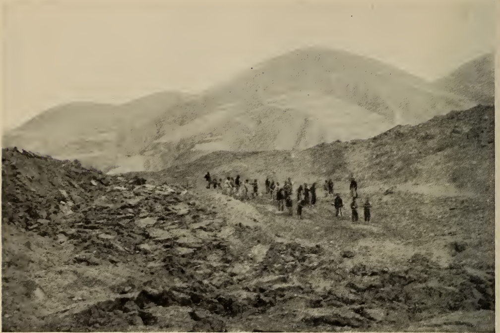
RELIEF WORKERS DIGGING TO RELEASE WATERS BEHIND A QUAKE-MADE DAM The earthquake made this dam of millions of tons of loose earth, stretching from valley-side to valley-side, in a few seconds of time.
