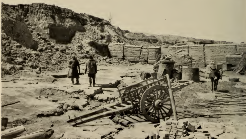
A THRESHING-FLOOR, ONCE LEVEL AS A DANCING FLOOR, CRACKED UP INTO MANY LEVELS BY THE QUAKE
