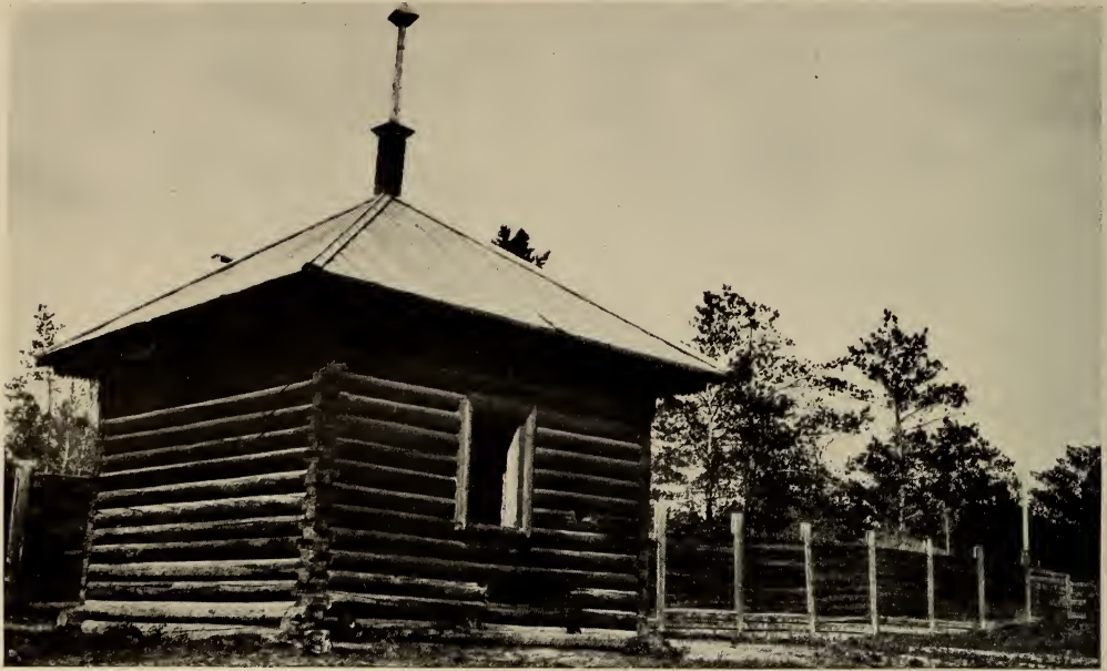
WELL-HOUSE AT SEMENOV'S CHITA HEADQUARTERS
