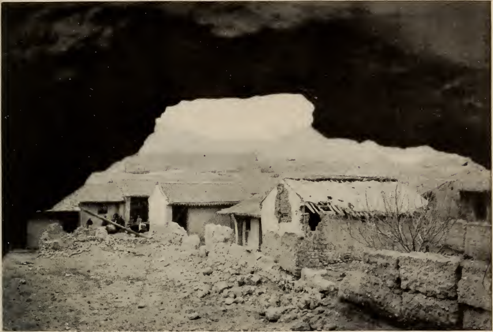
LOOKING INTO THE RUINED TOWN OF WATING THROUGH A HOLE SHAKEN THROUGH THE CITY WALL BUILT OF LOESS
