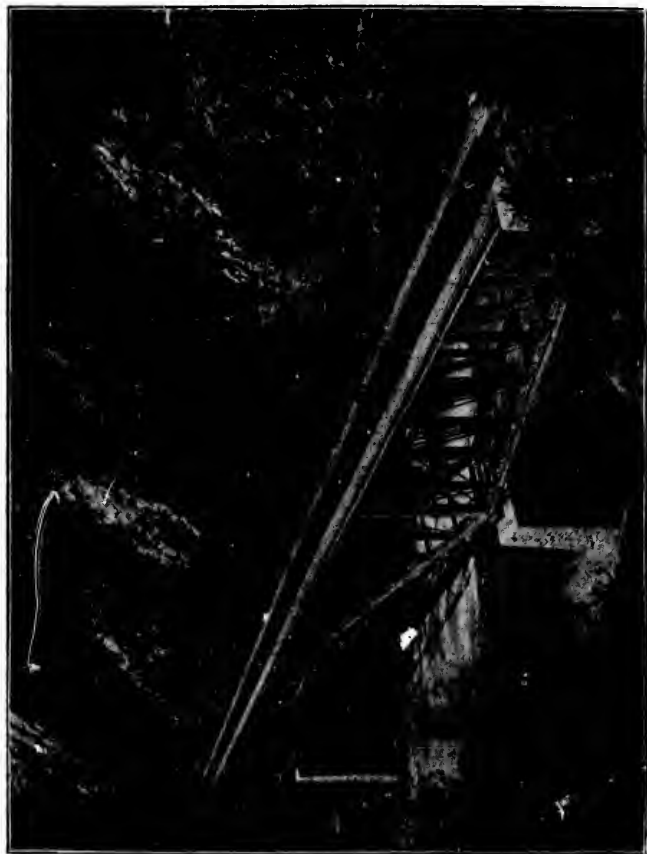
CANADIAN PACIFIC RAILWAY, CANTILEVER BRIDGE AT CISCO.
