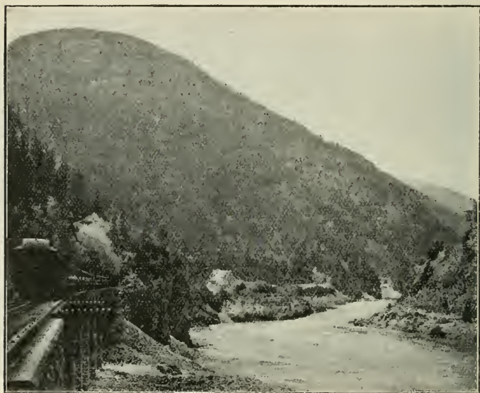
FOUR TUNNELS, FRASER CAÑON, BRITISH COLUMBIA.
