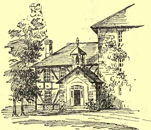
WING OF SHINGWAUK HOME.
