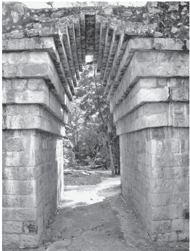
A fine example of a corbelled arch on the east flank of the Copán ball court. The Classic Maya never learned the art of the true arch, and thus interior rooms of stone structures were often small and narrow. (Courtesy of Janice Van Cleave)
