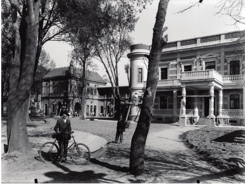
Plate 7 One unidentified person from the previous image appears again, suggesting that he is an engineer or architect directing construction. Fototeca Nacional del Instituto Nacional de Antropología e Historia.
