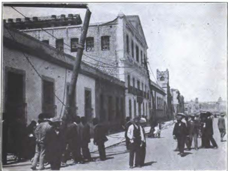
Iron telegraph pole smashed by shot from the arsenal
