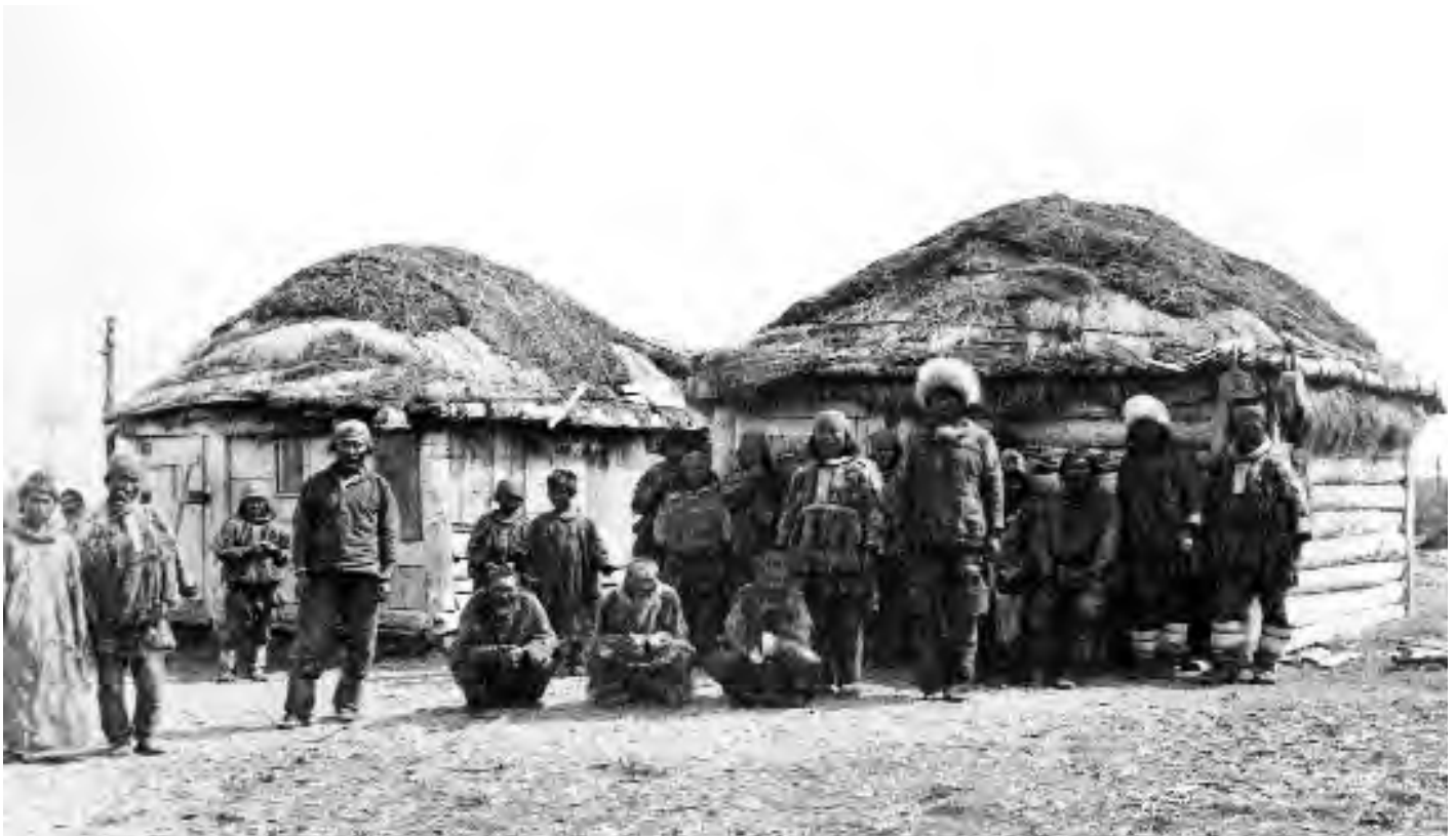
The Yup'ik created larger settlements in winter to take advantage of group subsistence activities. Villages ranged in size from two to more than a dozen houses, plus storehouses, such as this storehouse in Togiak, Alaska (1909).
