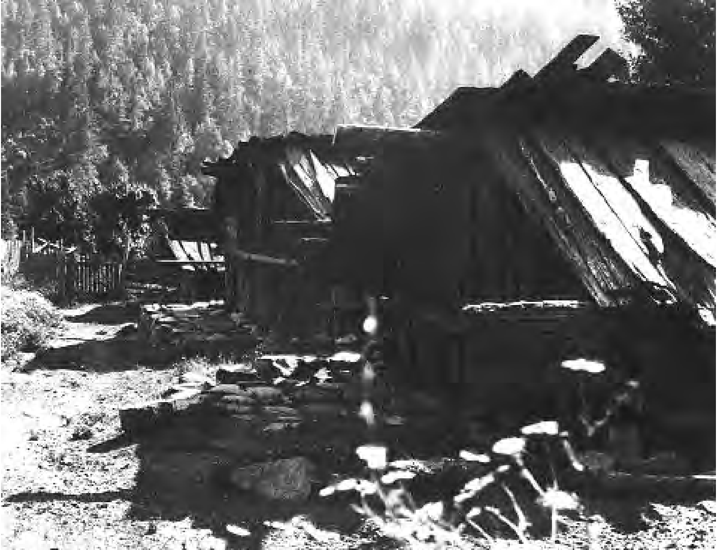
Yurok village dwellings, like the ones pictured in this 1890 photograph, were small rectangular redwood-plank houses with slanted or three-pitched roofs and a central excavated pit.
