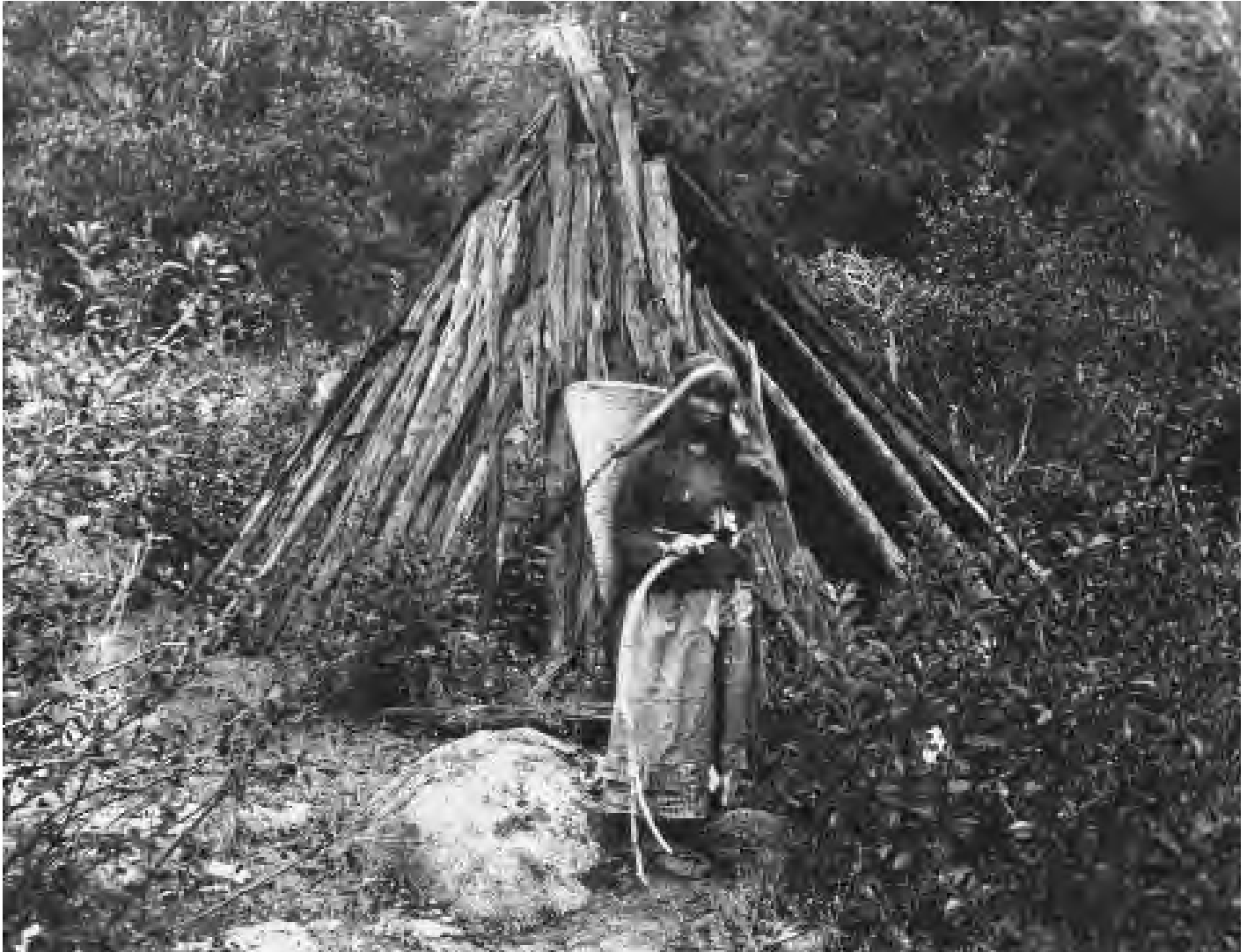
The Sierra Miwok and Mono peoples of the Sierra foothills built conical houses framed with wooden poles and covered with plants, fronds, bark, or grasses. Hearths were centrally located, next to an earth oven. Pine needles covered the floors; mats and skins were used for bedding. This photograph shows a woman in front of such a dwelling in 1870.
