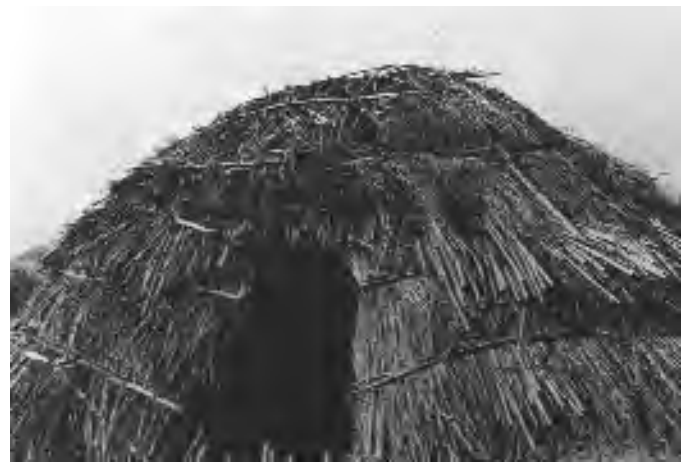
The Owens Valley Paiutes built several kinds of structures. Winter dwellings like this (early 1900s) were conical, semisubterranean, and built on a pole framework covered with tule, grass, and sometimes earth.
