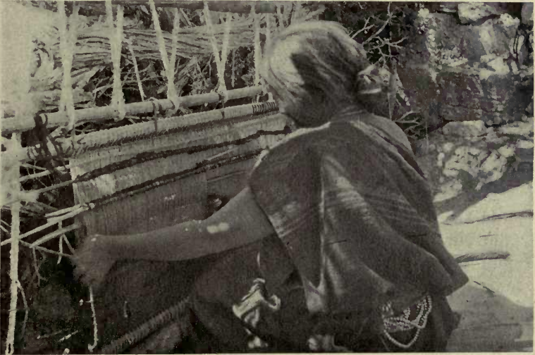
Fig. 21. Loom for weaving diagonal cloth.
