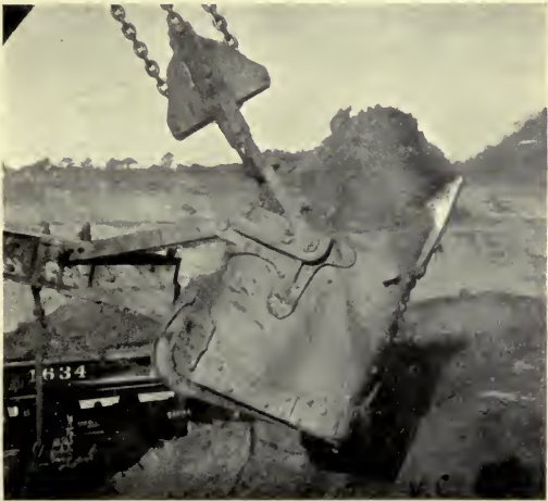
THE SHOVEL LOADED WITH SOIL.
