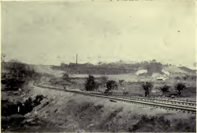
RE-LOCATION OF RAILWAY ABOVE GATUN.
