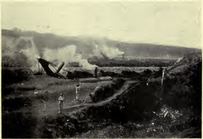
EXCAVATION FOR LOCKS, GATUN.
