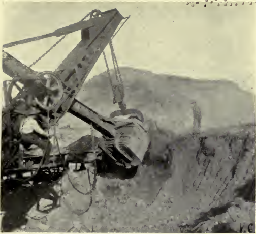
MARKS OF STEAM SHOVEL'S TEETH.
