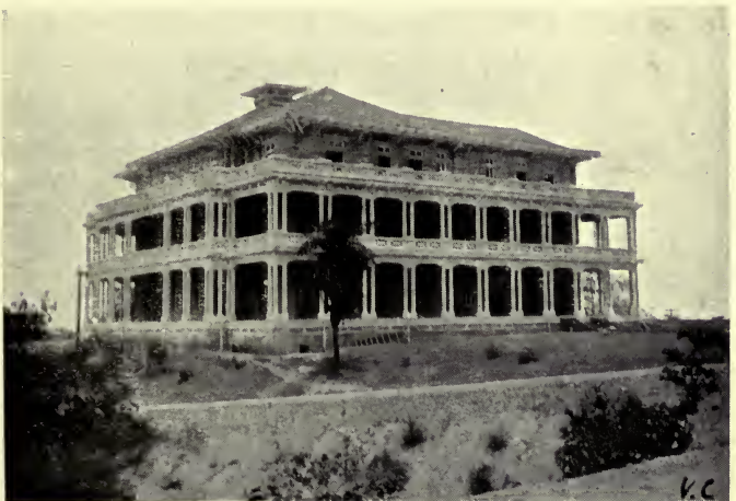
ADMINISTRATION BUILDING, ANCON.
