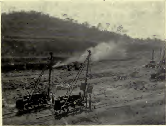
ROCK DRILLS IN THE CUT.
