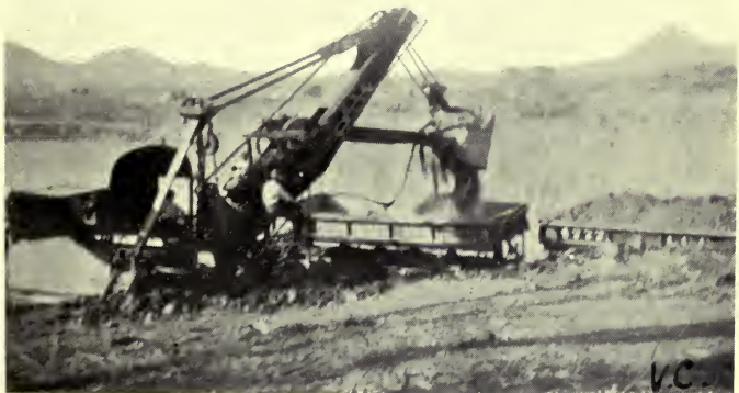
STEAM SHOVEL UNLOADING INTO DIRT CAR.
