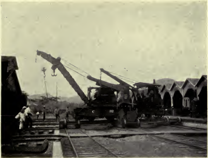
100-TON WRECKING CRANE, GORGONA.
