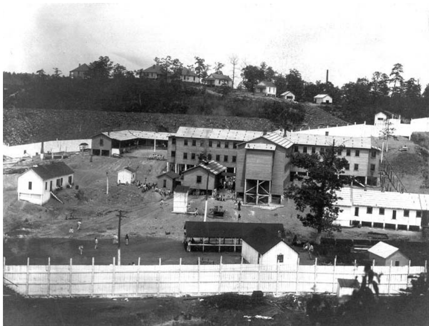
Banner Mine prison buildings that housed black convicts. (Courtesy of the Birmingham Public Library, Birmingham, Ala.)
