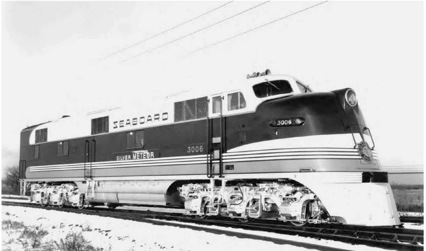
A builder's shot of Seboard E4A, No. 3006. EMC photo, author collection
