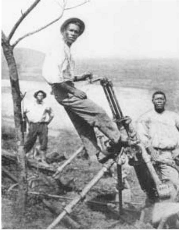
Three Jamaican men work with a compressed-air drill at Panama. The photograph is from Willis J. Abbott's Panama and the Canal in Picture and Prose, 1913. GENERAL RESEARCH AND REFERENCE DIVISION, SCHOMBURG CENTER FOR RESEARCH IN BLACK CULTURE, THE NEW YORK PUBLIC LIBRARY, ASTOR, LENOX AND TILDEN FOUNDATIONS.
