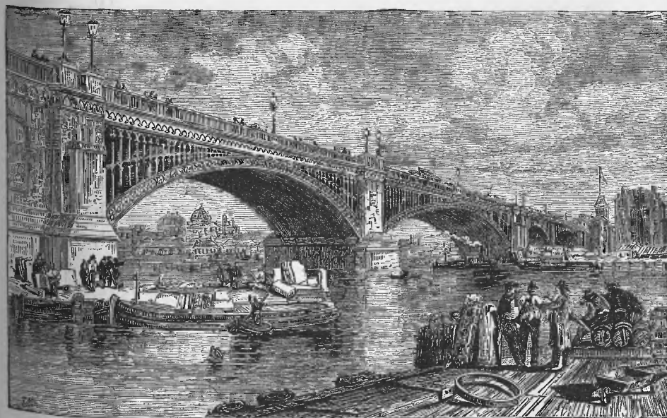
CHESTNUT STREET BRIDGE.
