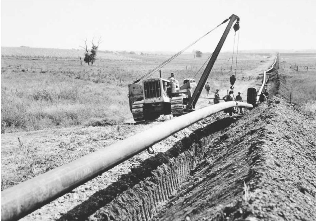
The Caterpillar Company specializes in heavy machinery built to perform specific tasks such as laying pipelines as shown here.
