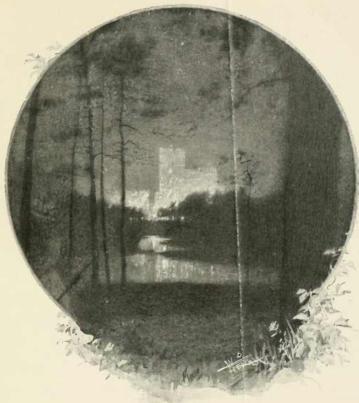
Hideous high buildings. Looking east from Central Park at night.
