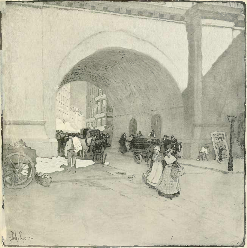
Under the Approach to Brooklyn Bridge.
