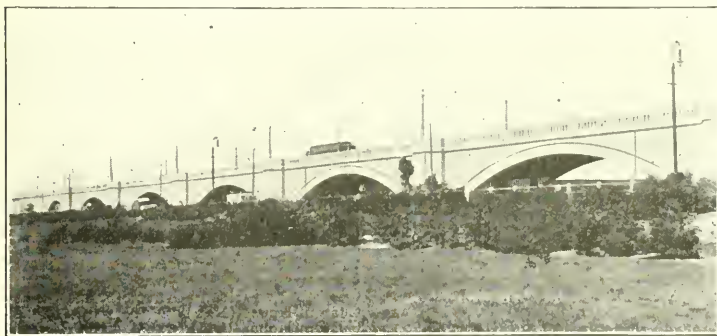
Charles River Dam and the Viaduct Page 50
