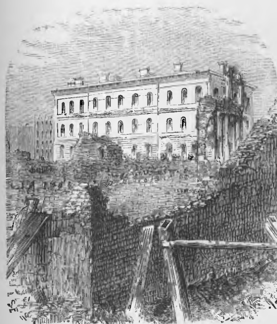
POST-OFFICE AND CUSTOM-HOUSE.
