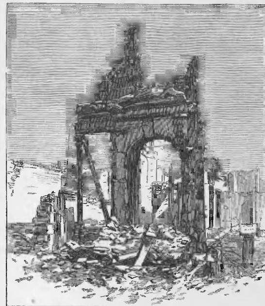
METHODIST CHURCH BLOCK.
