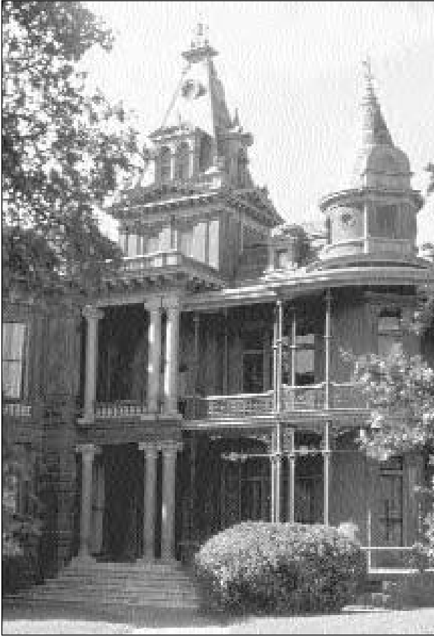
Cattle ranchers built great empires and fortunes, and these cattle barons built accordingly, as evidenced by the Littlefield House in Austin, Texas.
