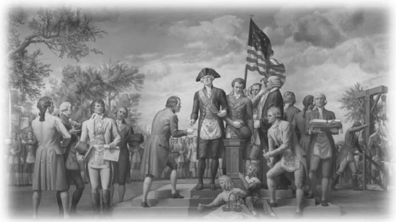
Allyn Cox's painting of Washington laying the cornerstone of the Capitol, September 18, 1793
