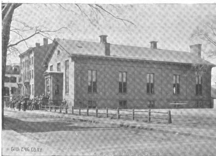
THE YALE DINING HALL BUILDING.
