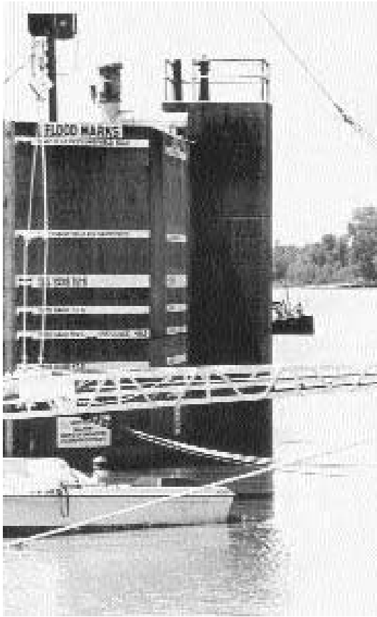
Mississippi River gauge at Vicksburg, Mississippi. Note the high level of the 1927 flood—"if levees had held." (Jesse Walker)
