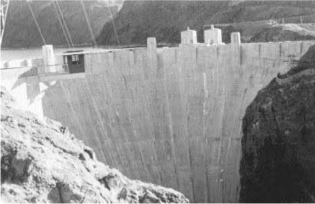
Hoover Dam (formerly Boulder Dam), a giant arch-type dam on the Colorado River completed in 1936 (Jesse Walker)
