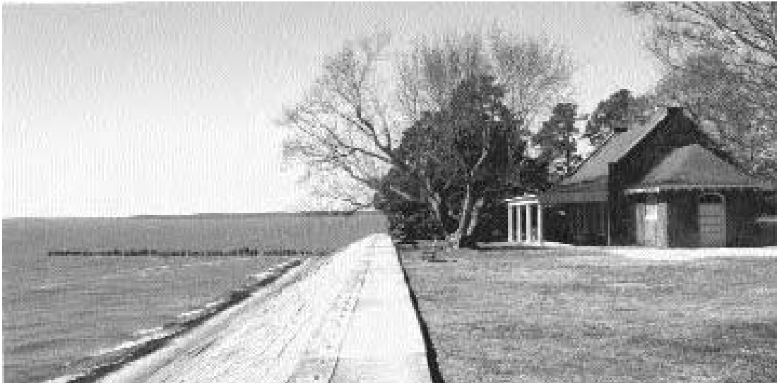
Seawall along the south side of Jamestown Island, Virginia, protecting the Jamestown historical site from erosion. The James River is to the left; the building to the right is used to process archaeological finds. (Laura Penn)
